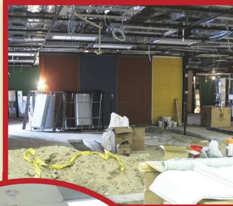
Mt. Vernon ES Remodeling of building B classrooms
