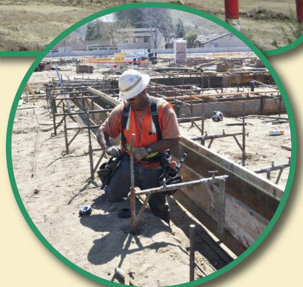
Little Mountain ES Setting up slab on grade for the Multi-use Building
