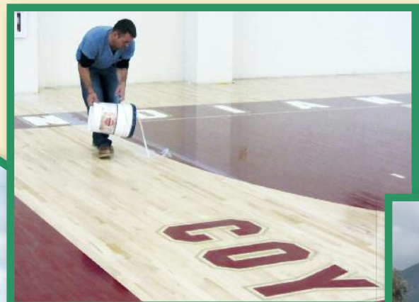
Indian Springs HS Sealing of the gym floor following striping
