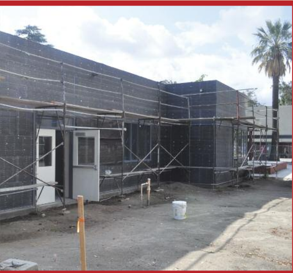
San Bernardino HS- Preparation for exterior plaster at Administration Building
