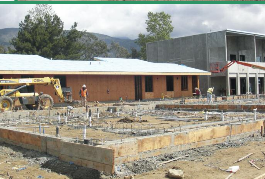
Little Mountain ES- Administration Building framing
