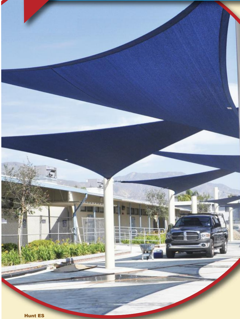
Hunt ES Work in progress for new lunch shelter area
