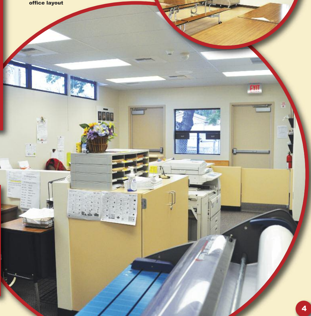
Inghram ES-Administration Office complete with new carpet, ceiling, lighting, paint and reconfigured office layout
