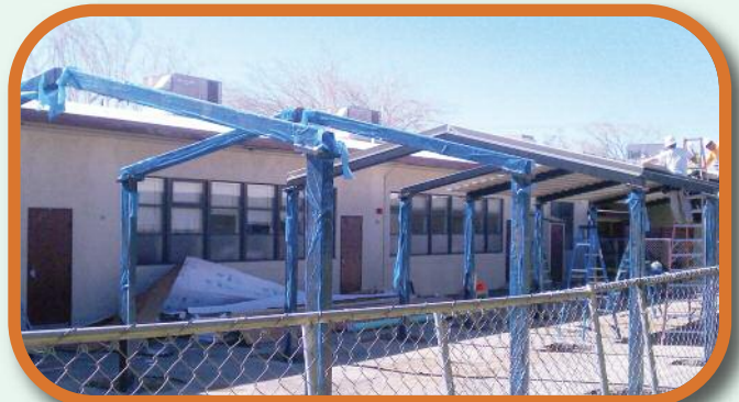
Hillside ES- New lunch shelter under construction
