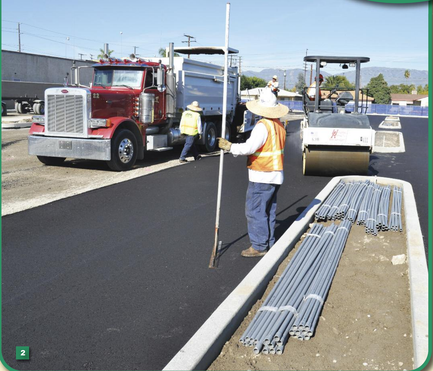
1 & 2- Middle College ES- Paving the parking lot
