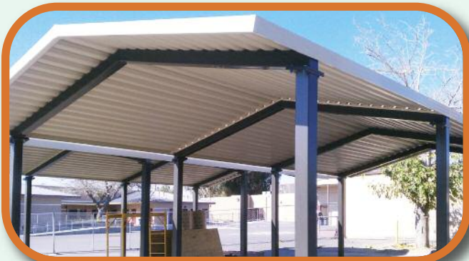
Roosevelt ES- New lunch shelter under construction
