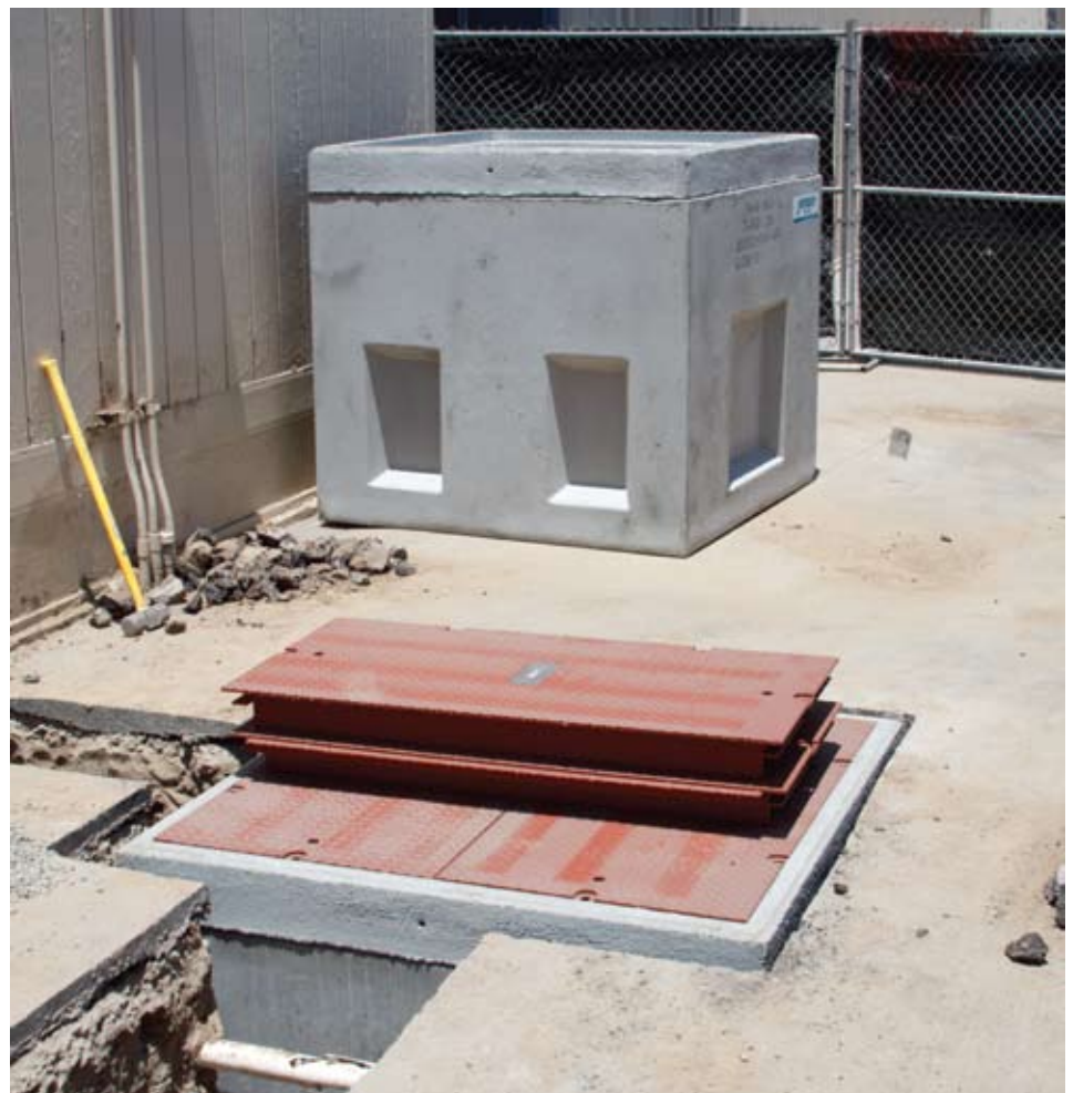
New electrical lines have been placed at Hunt ES to support a relocated teacher’s lounge and library.
