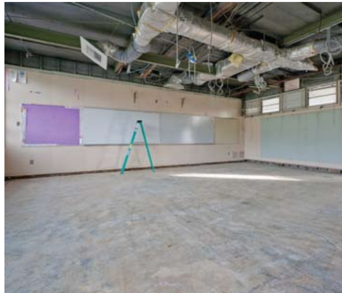
Hillside ES Old flooring and ceiling systems have been removed from this classroom. The HVAC system is in good condition and will remain.
