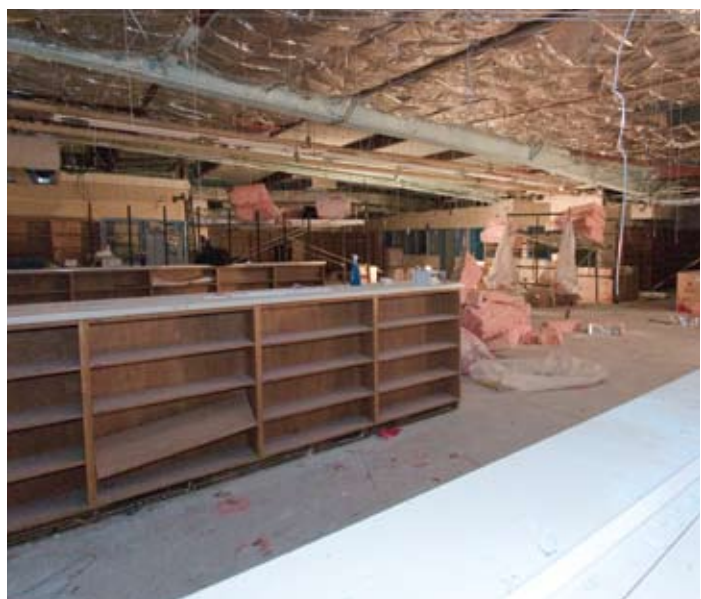
Inside the library, old wallpaper has been removed from the walls. New insulation has been placed in the ceiling.
