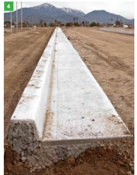
1 Workers pouring concrete for the exterior wall base that will be part of a new music building. Part of the ground has been excavated to make room for a choir room. 2 & 3 Additional trenches have been dug between the existing buildings where additional utility lines will be installed. 4 Concrete curbs are established in the new parking and the track & field areas.
