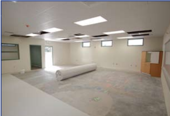
Casework installation is nearly completed; carpeting and flooring is about to begin.
