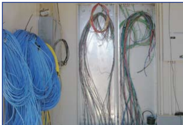
Electrical and data wiring are being pulled throughout the building and will be punched into the electrical room.
