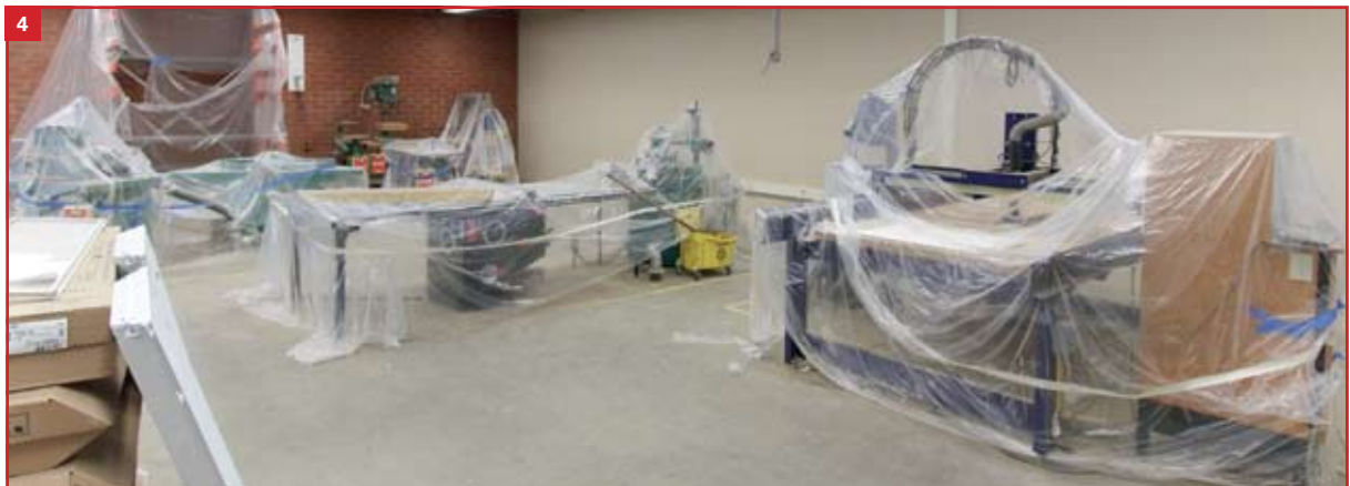
4 Work continues in Building E. In this room, equipment for a wood shop class has been covered up while the room receives a new coat of paint. Electrical, lighting, and public announcement systems have also been upgraded. 5 ADA-compliant ramps installed along Building G. A new ramp has also been constructed at the swimming pool area (not pictured).
