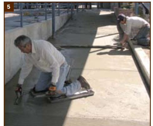
3 A worker digging a utility trench at the High School #8 site. 4 One of four new SDC buildings completed during the past year, this building at Hunt Elementary School is now serving as temporary housing while modernization work begins. 5 Workers completing a ramp and paths of travel at Fairfax Elementary School in March 2009.
