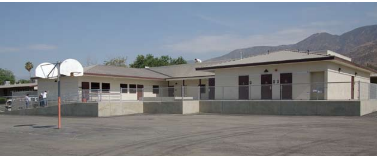
Hillside ES: As modernization projects progress at both campuses, classes were moved into the recently completed SDC buildings to vacate classrooms for interim housing relocations.
