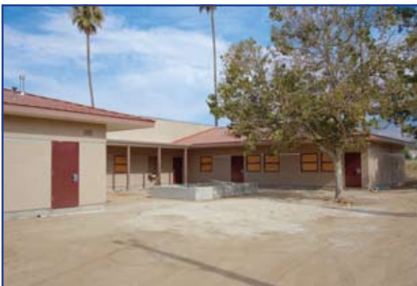
The surrounding areas has been prepped for concrete and asphalt pouring.
