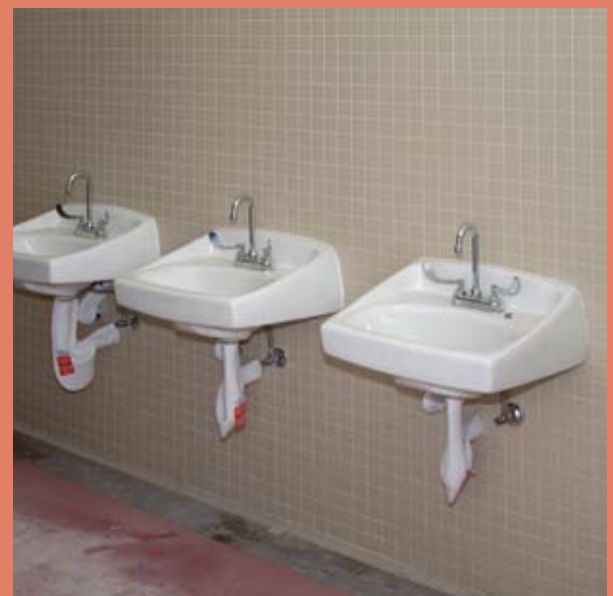
Warm Springs ES: Existing restrooms at both locations have been renovated to meet federal ADA standards.
