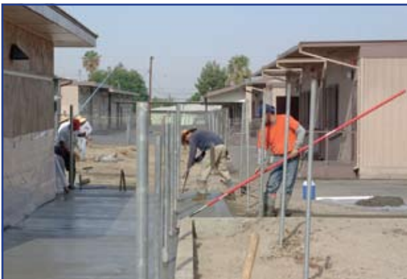
Workers pouring and laying out concrete sidewalks around the building.
