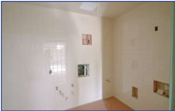
Tile work on the walls are finished in the restrooms; flooring and fixtures to follow.
