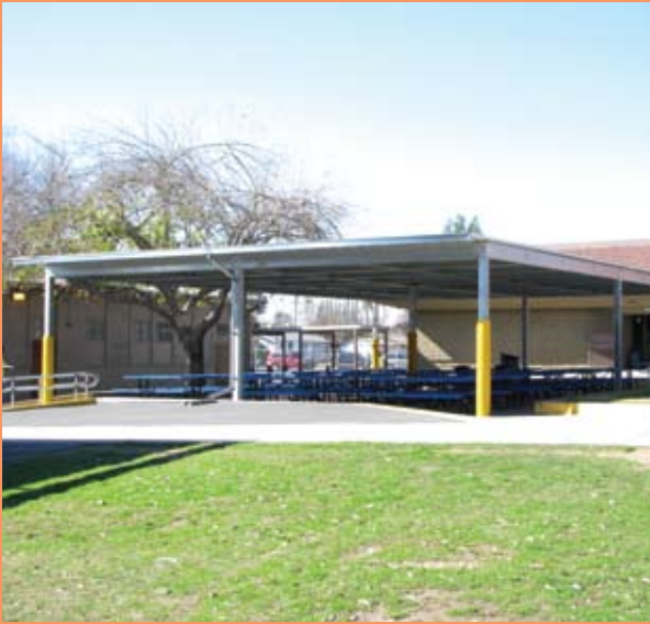
The Mt. Vernon lunch shelter will provide protection to students from the sun and rain.
