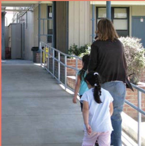
Fairfax ES: New ramps and paths of travel have been built throughout both campuses.
