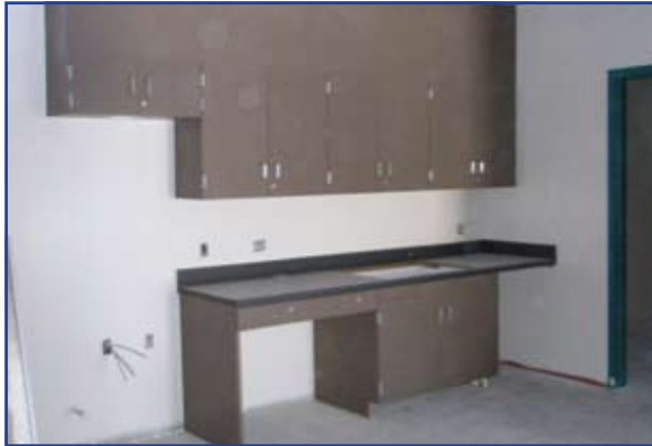
Casework is installed and electrical wires are being pulled.
