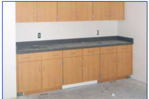
Casework has been installed throughout the building. Finish electrical and plumbing work has started.
