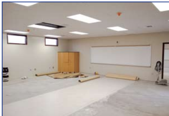
Progress continues inside with casework and flooring.
