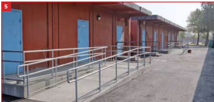
4 Work continues in Building E. In this room, equipment for a wood shop class has been covered up while the room receives a new coat of paint. Electrical, lighting, and public announcement systems have also been upgraded. 5 ADA-compliant ramps installed along Building G. A new ramp has also been constructed at the swimming pool area (not pictured).
