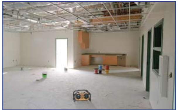
Casework and the ceiling grid are complete. Data and electrical wiring are being pulled throughout the building.
