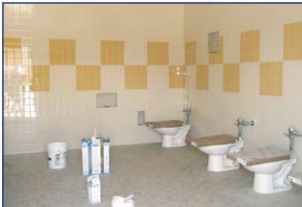
Finish work in the restrooms has begun. Toilets in this restroom have been set.
