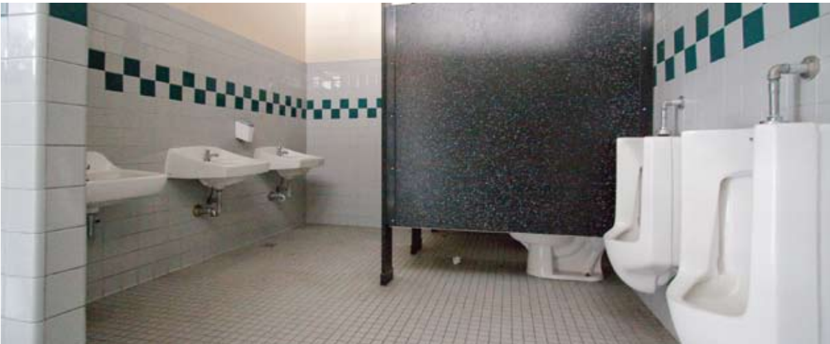
Hunt ES: The restrooms at both campuses will be completely renovated in order to comply with federal ADA requirements.
