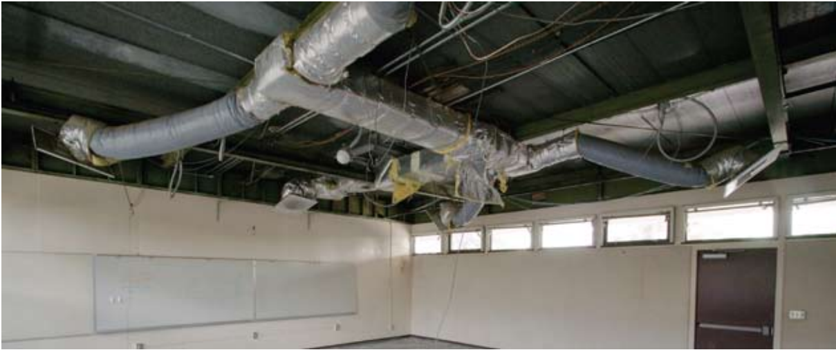
Hillside ES: At both sites, the HVAC duct work remains in good condition. This will result in a savings that will be reinvested for additional work.
