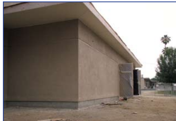
The final coats of paint have been applied to the exterior of the building. At every site, the layers of stucco and paint are the same color to reduce visible signs of wear.
