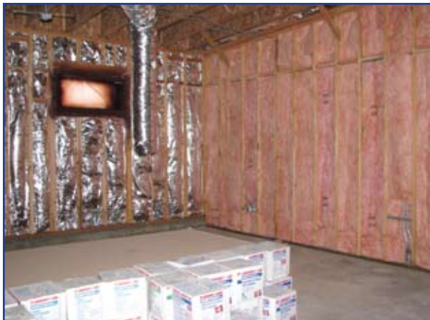
Insulation and sheetrock installation progresses; elsewhere, tile work is underway with scratch layer installation.
