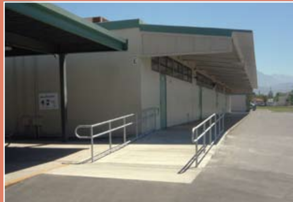
Warm Springs ES New ramps installed. Restrooms also completely renovated.
