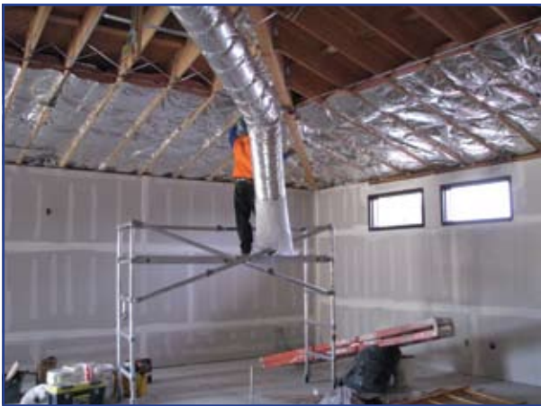
An installer applies insulation to the interior roof.
