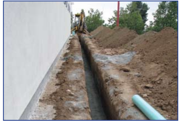
Trenching for a storm drain line alongside the building. The line will help drain water that can pool at the top to the bottom elevation.
