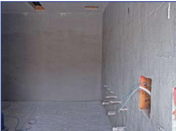
The second "scratch" layer applied to the walls of the restrooms where tile installation has started.
