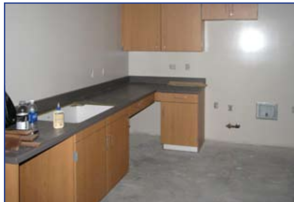
Painting, casework installation, plumbing fixtures, and electrical are in the process of installation.
