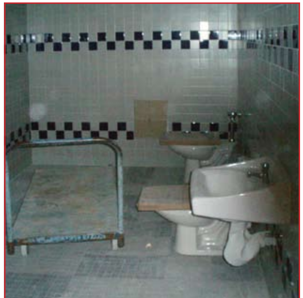
Final work inside restrooms includes installation of finish fixtures and stalls.
