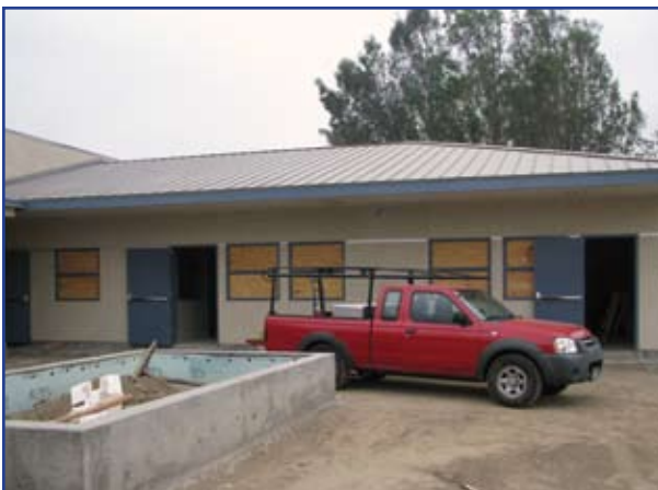
With construction nearing completion, windows are boarded to protect against vandalism.
