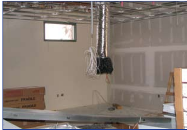
Electrical wire strung throughout the building. Sheetrock and insulation have also been installed.
