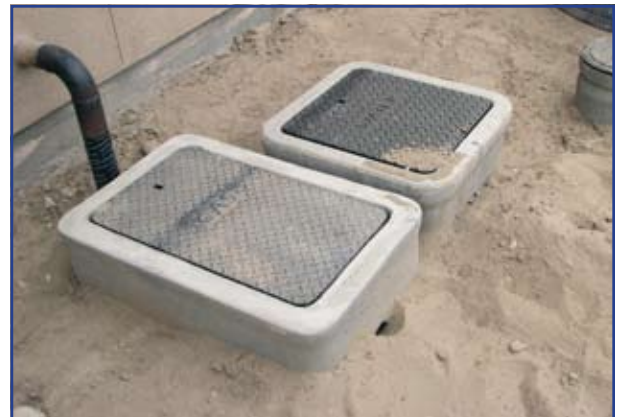
Utility meters placed next to the building. All utility lines at the SDC building are connected to the main campus lines.
