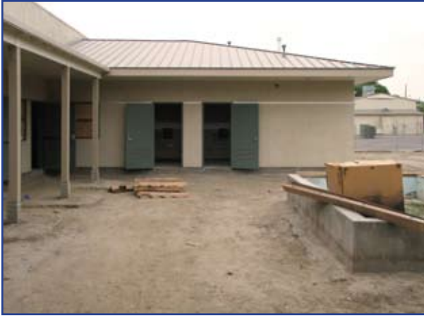
Exterior finishwork is nearly complete. The surrounding areas are graded for asphalt and concrete.
