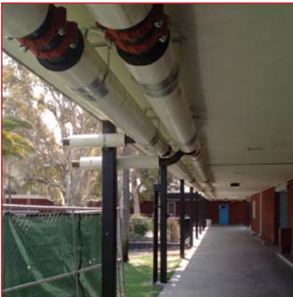
Special hydronic pipes used for heating and air conditioning are installed and insulated.
