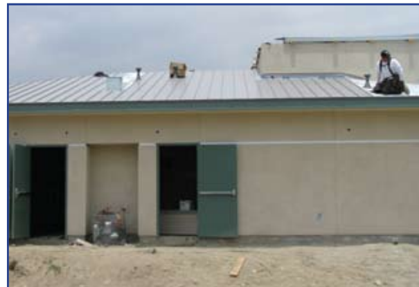
A roofer installs the last of the roof shingles on one section of the building.
