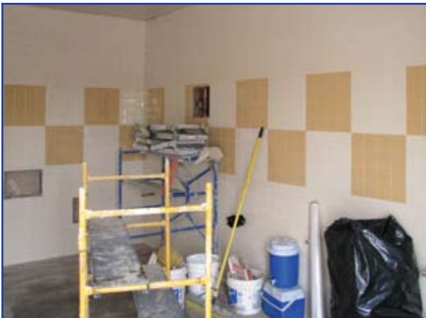
Wall tiling work in restrooms completed; finish fixtures and flooring to be installed next.
