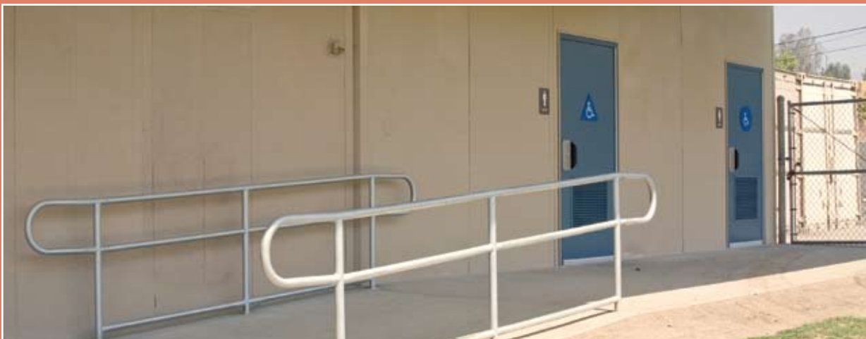
Fairfax ES A newly constructed ramp leads to the renovated restrooms, which allows easier access to the facilities.
