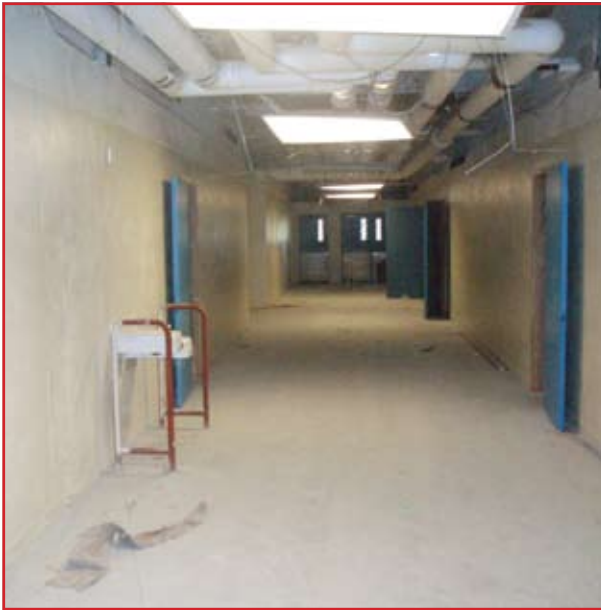
Ceilings and flooring are all that remain in the interior of Building C. A coat of paint has been applied to the walls.
