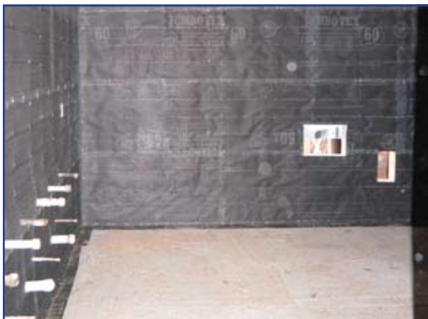
Lath layer applied inside restroom areas prior to tiling. Insulation and drywall have also been installed throughout the inside.
