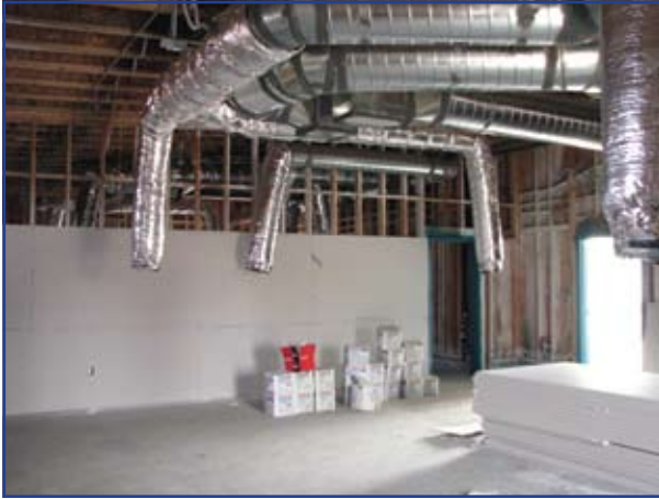
Sheetrock and insulation currently being installed on the interior walls of the building.
