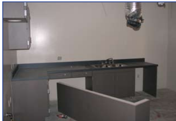
Casework installation started. Here, a work area equipped with a sink is being built; walls painted.
