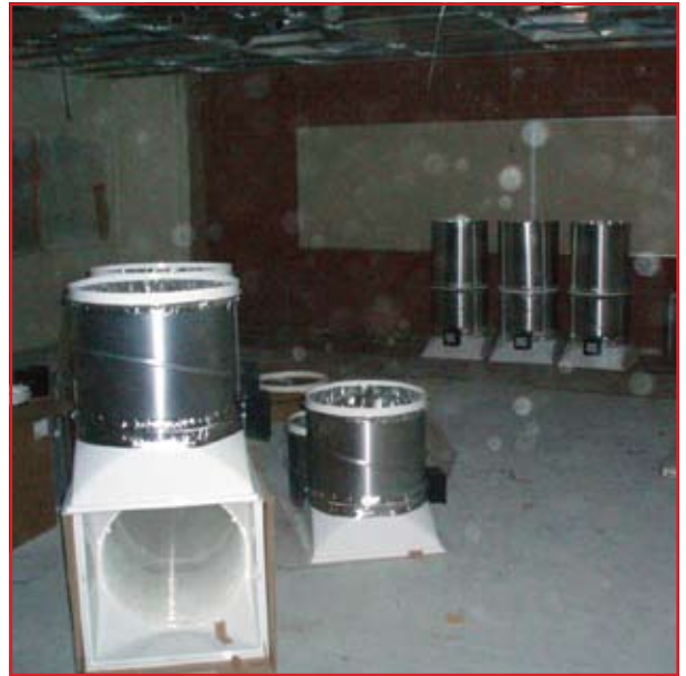
HVAC duct work awaiting to be installed inside a classroom in Building C.
