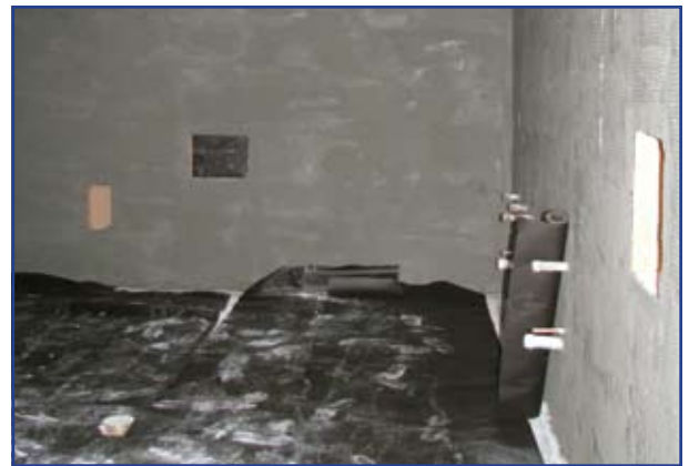
The second layer, a scratch coat, is applied to the floor and walls of the restrooms prior to tile installation.
