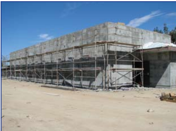
Stucco has been applied to the outside of the building; the final color coat to be applied next. Interior plumbing and electrical conduit going in. Exhaust fans delivered and installed
