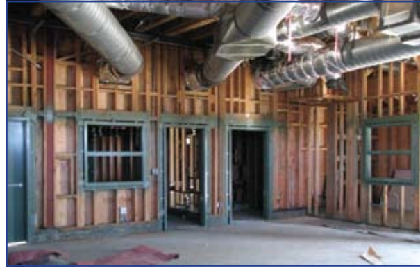
Progress continues inside as duct work, electrical, and door & window frames are installed.
