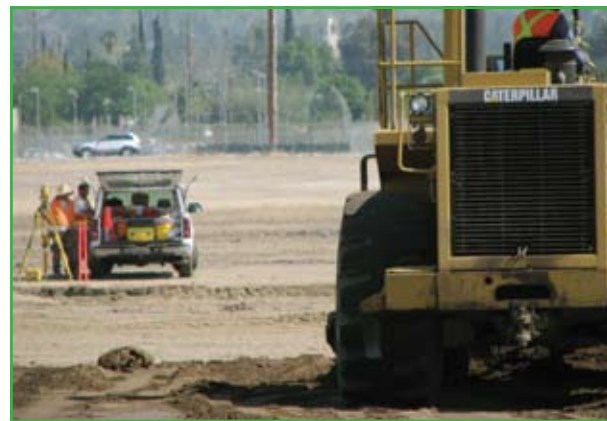
Meanwhile, surveying and grading continues on the remainder of the campus where new buildings and track will be built.
