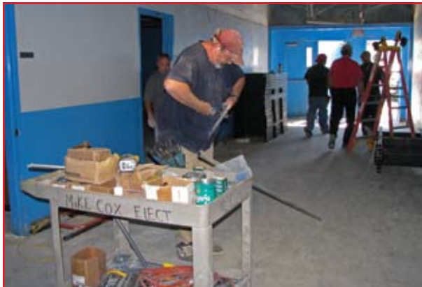
Electricians working on upgrading the electrical systems throughout the campus.
