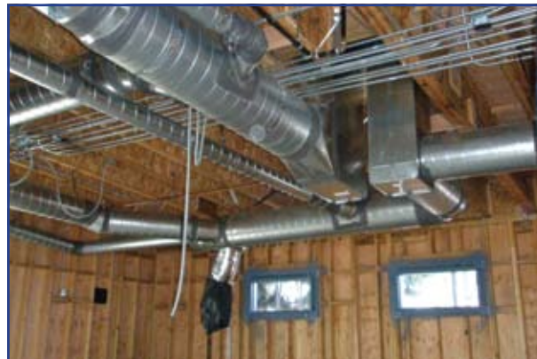
HVAC ductwork connected to HVAC units; openings framed, sheetrock to go up on walls next.
