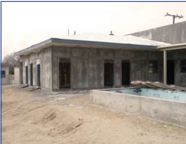
Exterior view of building with stucco and roof work ongoing.
