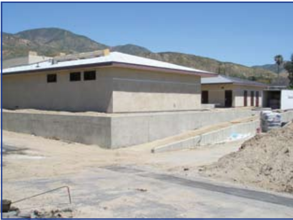
A fresh coat of paint has been applied to the exterior of the building.
