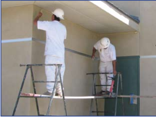
Workers applying paint to the exterior of the building.
