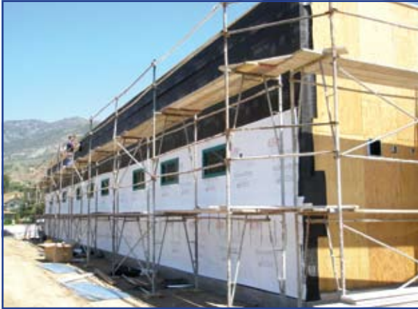
Scaffolding is erected as stucco work commences. A water-resistant membrane is being applied first.
