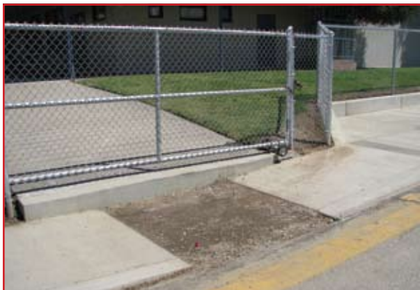
Fairfax ES A sidewalk on campus being upgraded for ADA-compliance.
