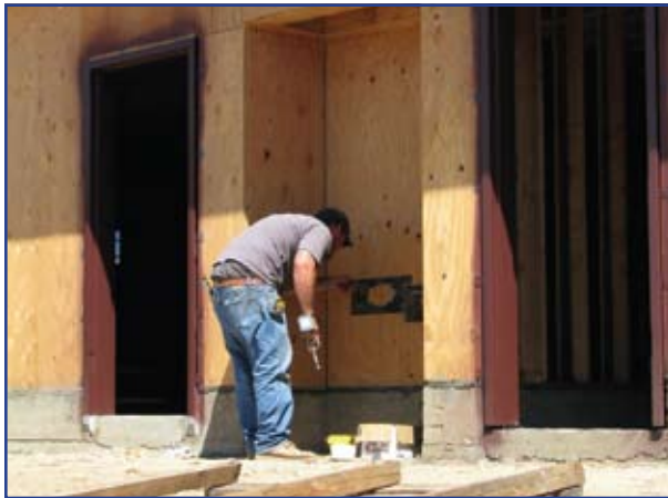
A worker is installing the wall mounts for new drinking fountains.
