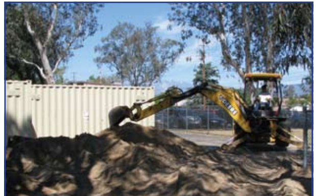
Trench work for sewer connection is dug up alongside the building.
