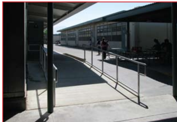
Warm Springs ES An ADA-compliant ramp has been completed; staff restroom upgrades under construction.
