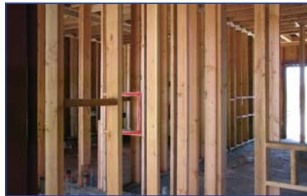
Inside, rough framework has been completed and plumbing and duct work will begin.
