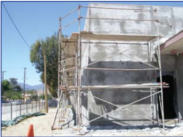
The third "scratch" coat is allowed to dry as part of the 5-step stucco process.
