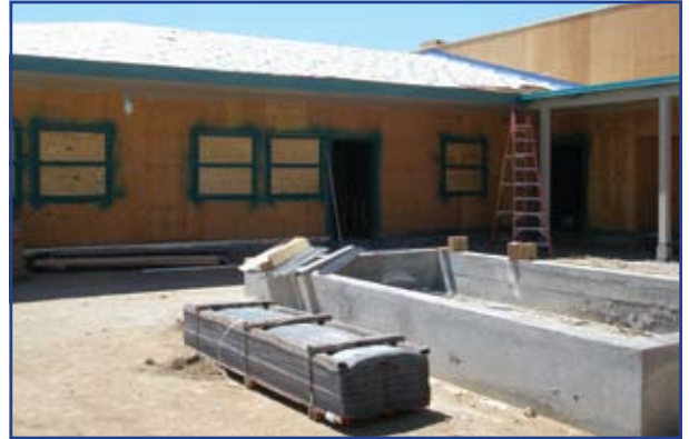
Steel door and window frames have been recently installed and prime painted; roofing sub-membrane is being installed.
