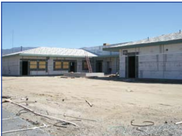
Water-resistant membrane and metal lath installed to the building's exterior.
