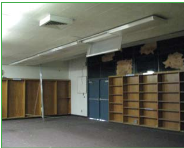
Inside the existing buildings, demolition and abatement work continues. This photo was taken in the old library.
