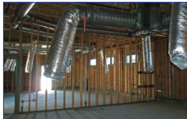
HVAC system flexduct installed; to be connected to exhaust vents after ceiling is hung.
