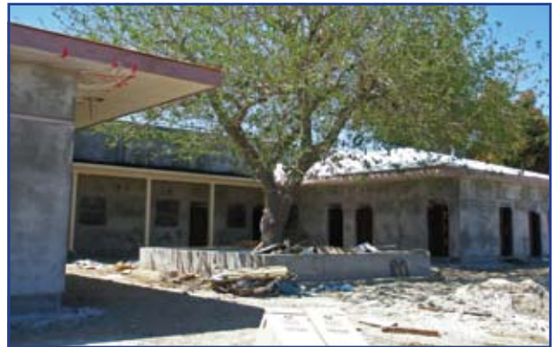
View of the "courtyard" with mature tree from original site landscape with plumbing and electrical roughed in the exterior!
