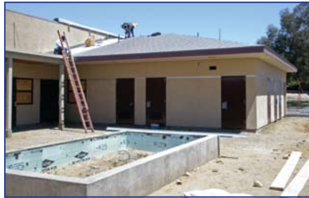
Workers also applying the final touches to the roof. New doors and windows have also been installed.
