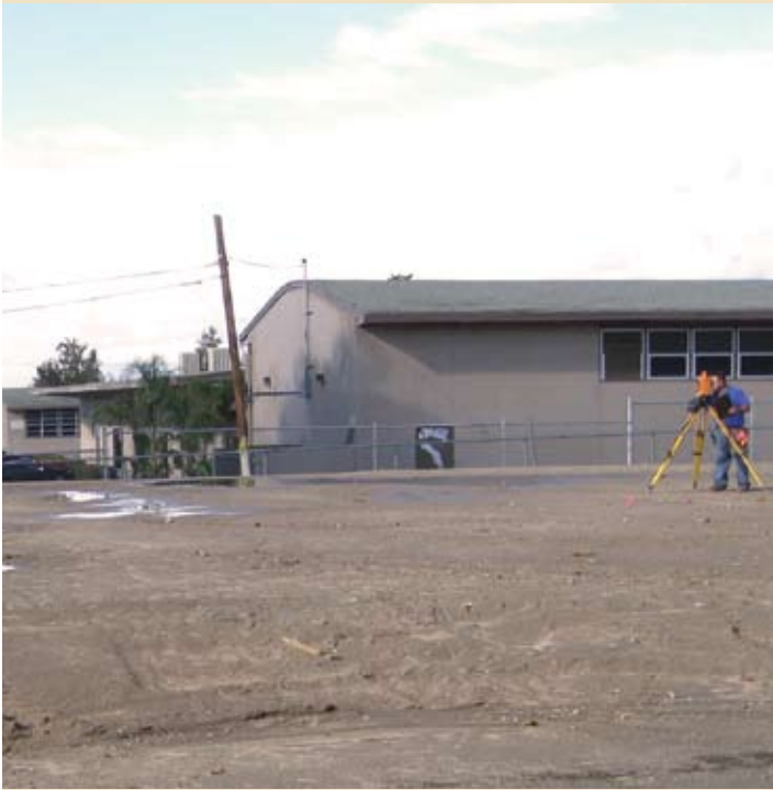
Initial site survey kicks off construction.
