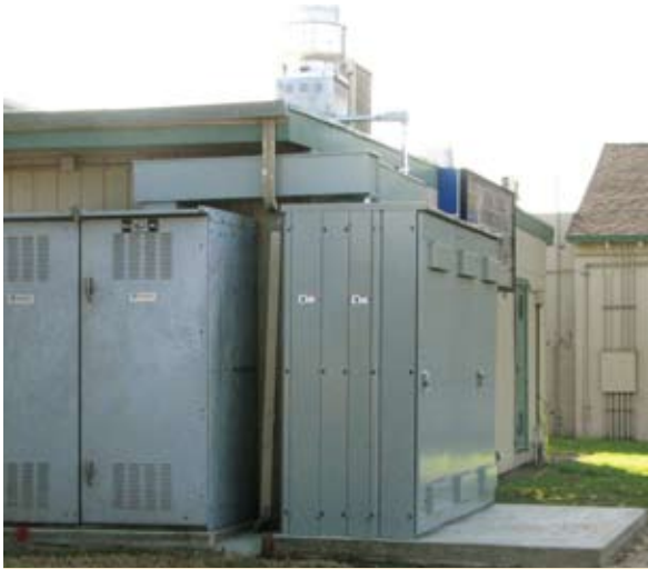
New electrical panels installed for upcoming system upgrades to classrooms.
