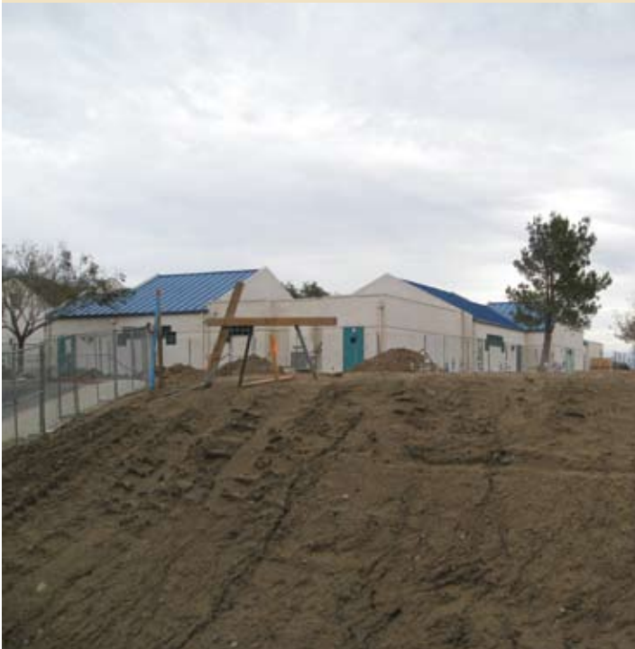
Grading at this site involved import of 13,000 cubic yards of earth to build up site elevation.
