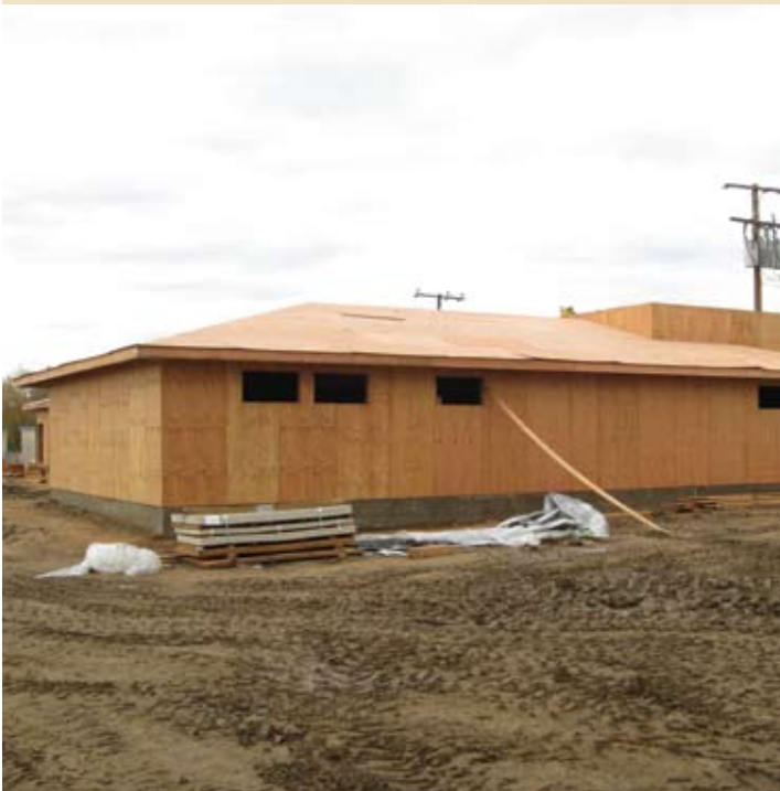
Structure enclosed; exterior siding is next while interior utilities are being installed.
