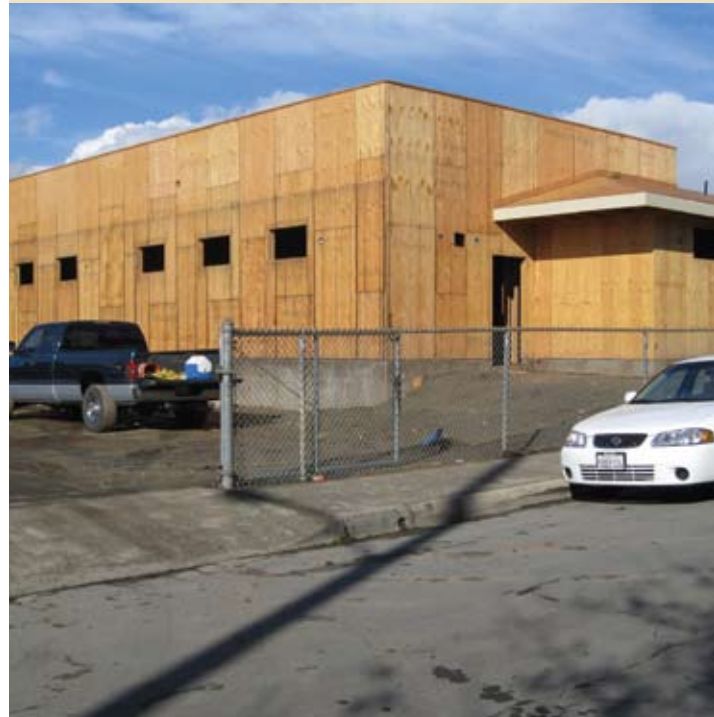
Structure framed and enclosed, ready for application of water-resistant membrane to exterior; interior electrical and plumbing is underway.
