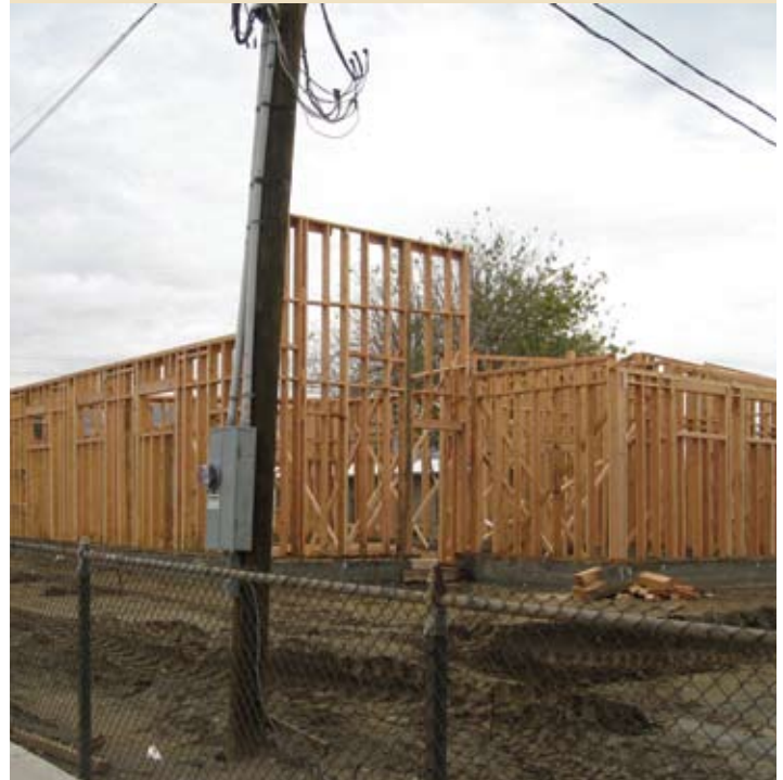
With the foundation concrete cured; structural framing is underway.
