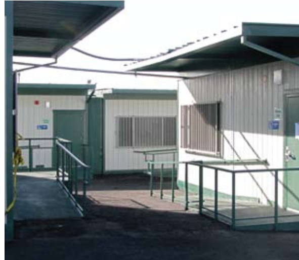
Students and teachers relocated to interim housing with entrance ramps and electrical completed.
