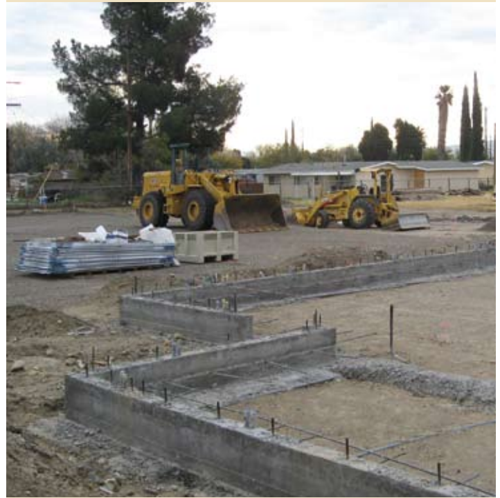
After site graded; foundation concrete is poured.
