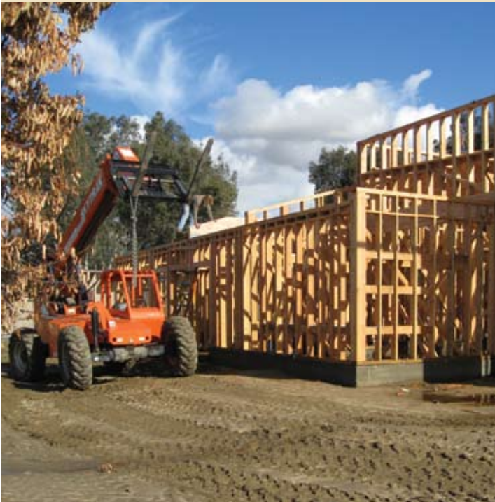
As framing continues, roofing materials are placed on top of building.
