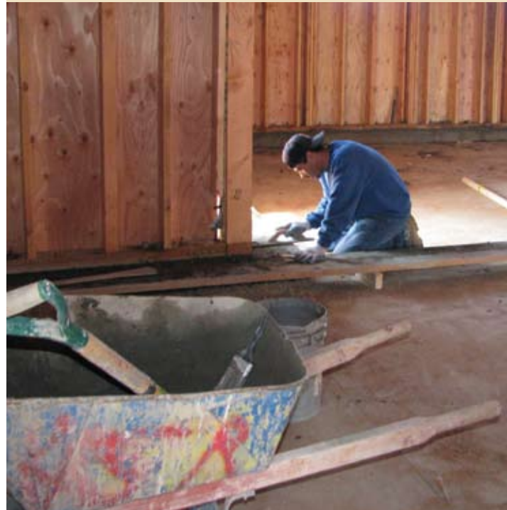
Concrete foundation rough finishwork for structural tie-ins continues.
