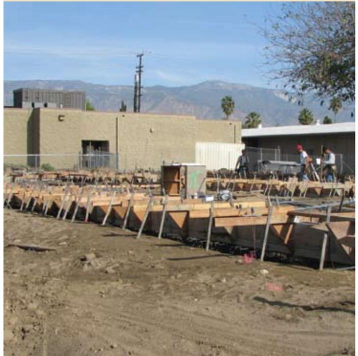
Foundation pad formwork and rebar in place for concrete pour.
