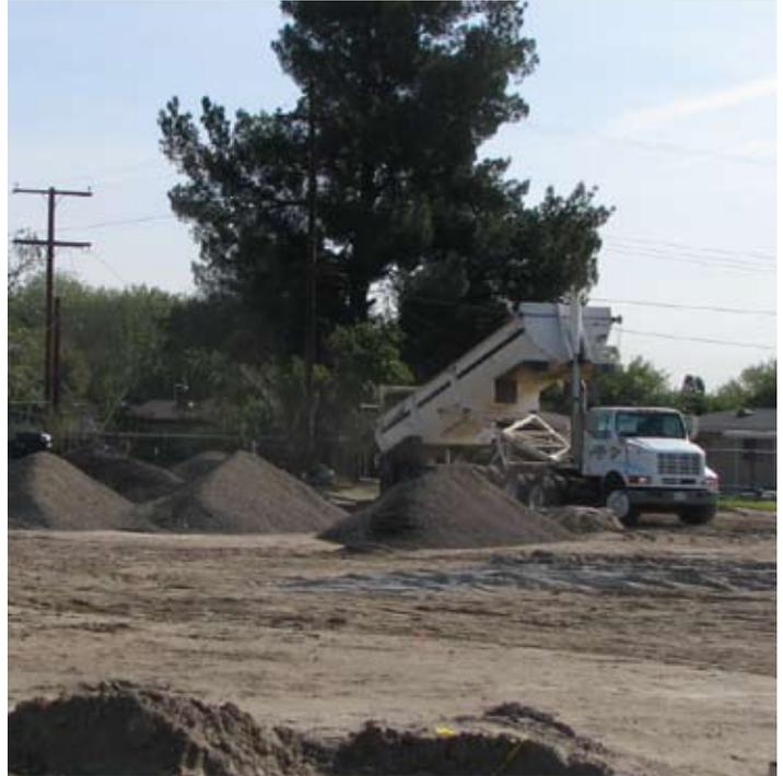
Underground utilities stubbed out and back filled; formwork and concrete for foundation pad are next.
