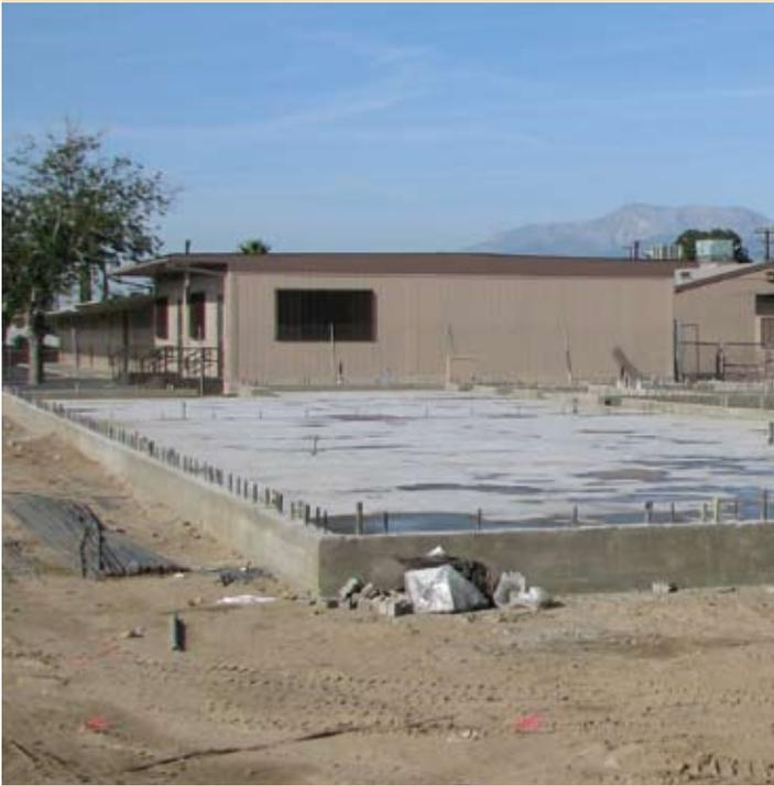
Concrete foundation pad poured, framing to start.
