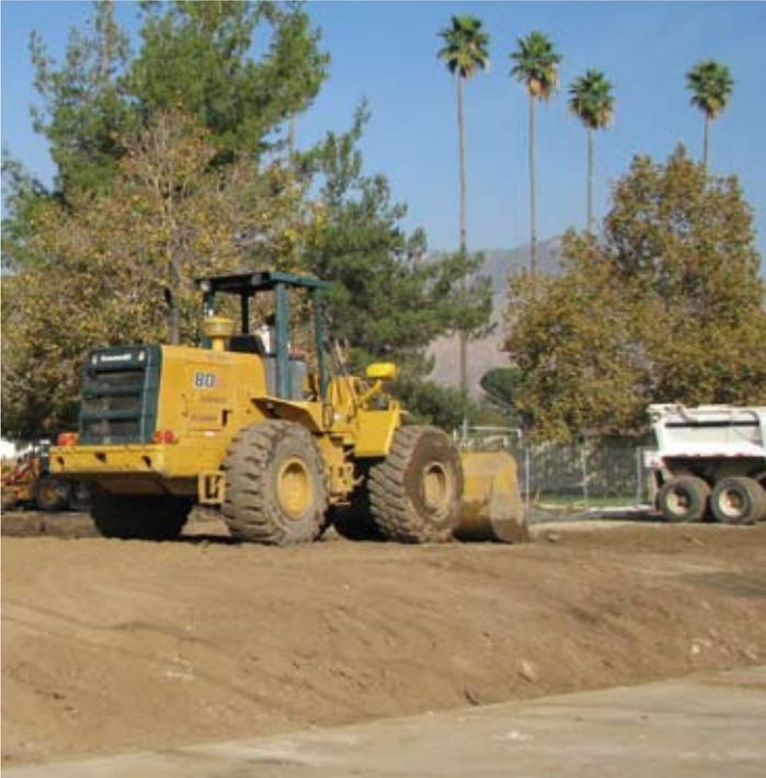
Sitework is underway with earthwork and demolition of existing concrete parking slab.
