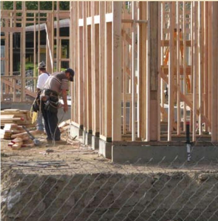
Structural framework going up and will be enclosed with plywood siding and roofing.
