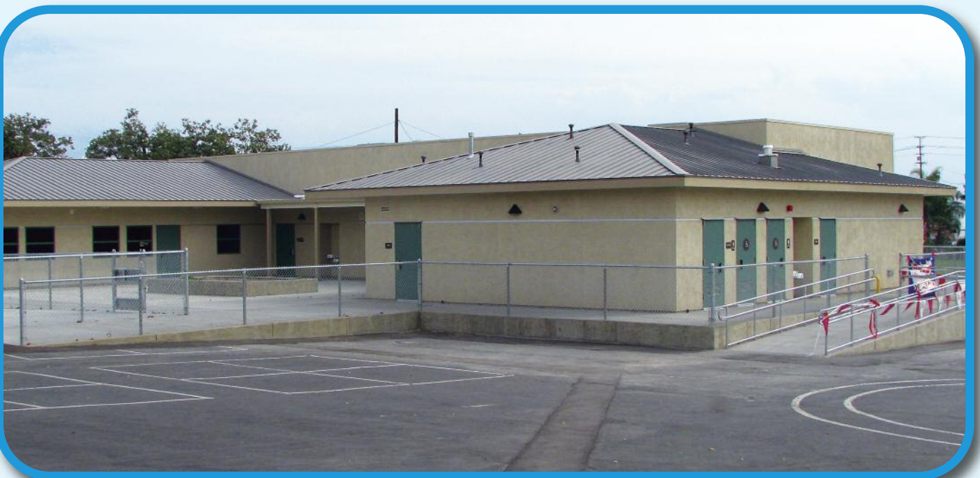
Bradley ES- Completed SDC Building
