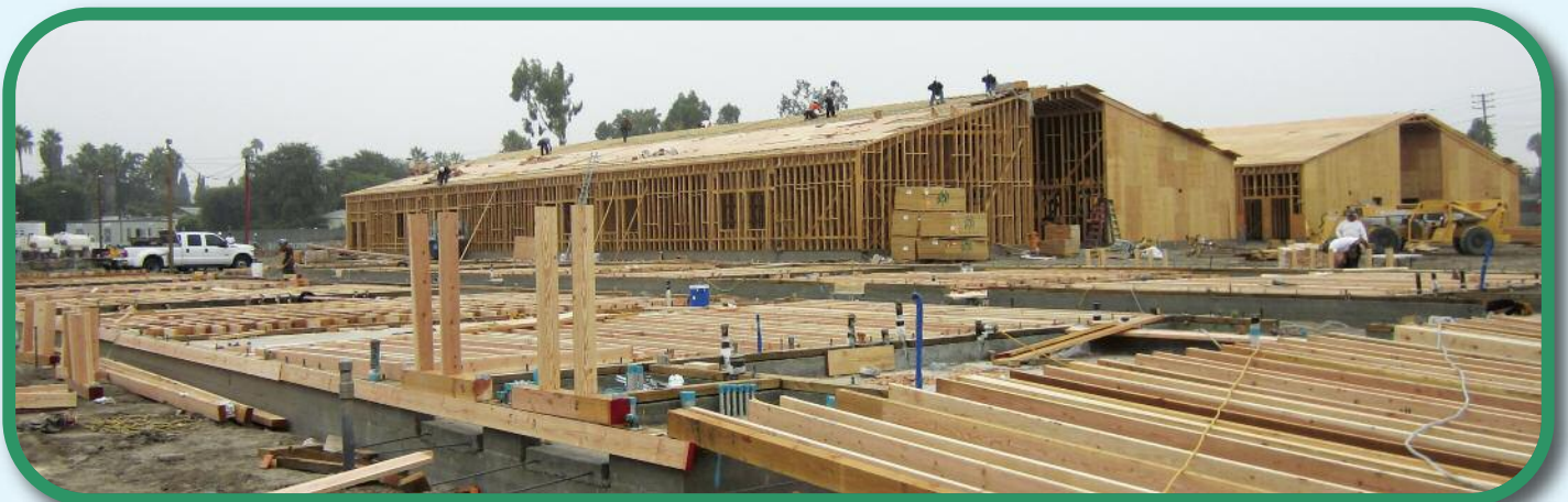
Captain Leland F. Norton ES- Building 4 framing under construction
