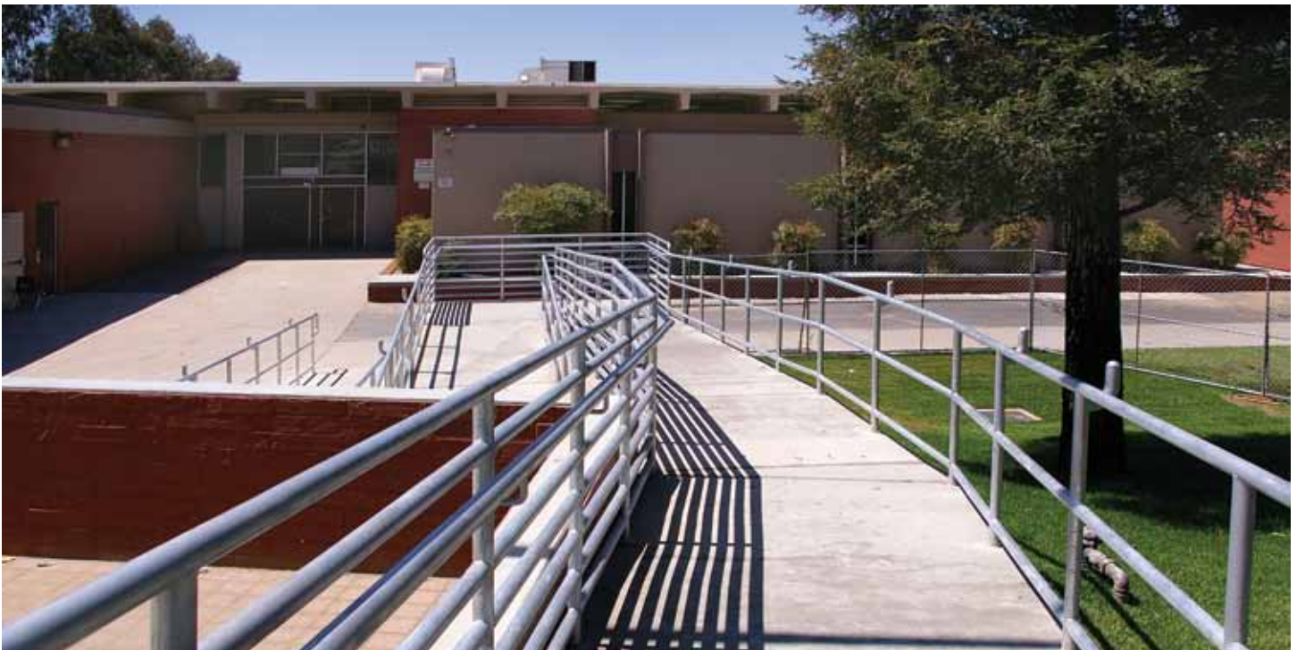
Serrano Middle School: Modernization
