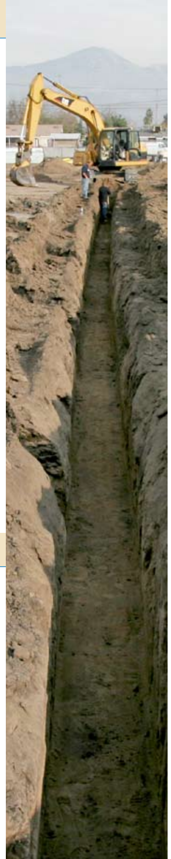
New campus Wong Elementary School trenchwork.
