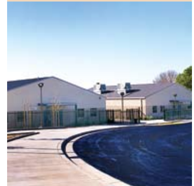
Rodriguez Prep Academy New Campus Classroom Buildings D and C from north campus bus and vehicle area.
