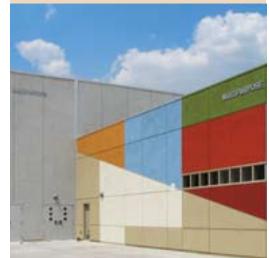
Curtis Middle School New Campus Rear view of the new Multipurpose Room.
