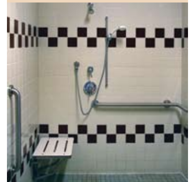
Del Vallejo Middle School SDC Classroom Fully ADA accessible showers are included in all SDC buildings.
