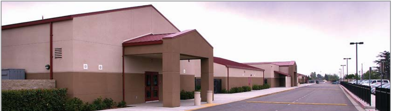
Anton Elementary School New Campus Administration Building
