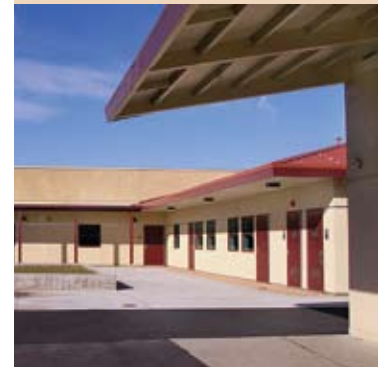
Golden Valley Middle School SDC Classroom SDC classrooms tie into existing campus walkways.
