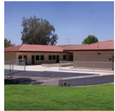
Serrano Middle School SDC Classroom Exterior view featuring fencing and landscaping.
