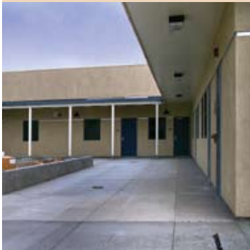
San Bernardino High School SDC Classroom Interior covered courtyard
