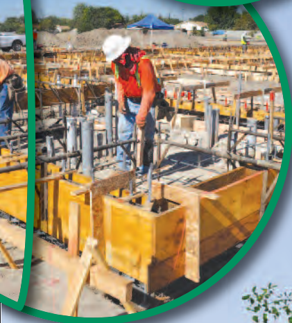
Graciano Gomez ES Construction of forms for footings
