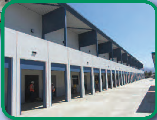
Little Mountain ES Two story concrete classroom building
