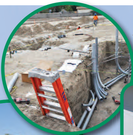
Graciano Gomez ES Site underground electrical
