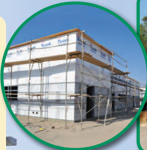
George Brown ES Classroom Building B1 lath
