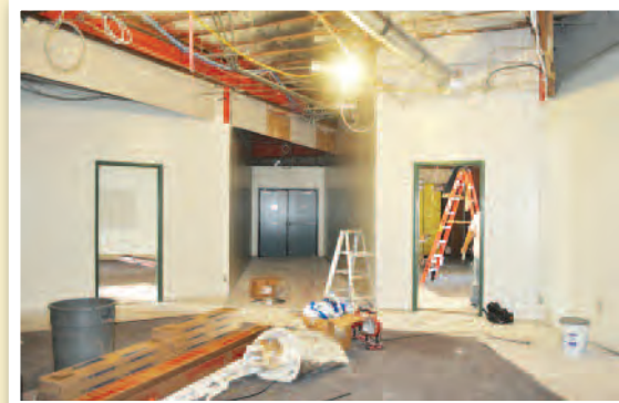
Bradley ES- Building M air conditioning and electrical work during construction
