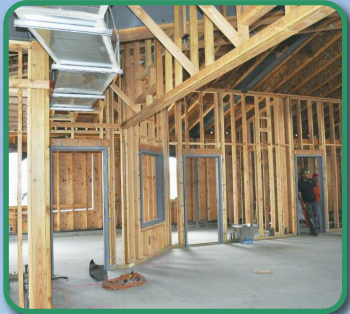
Middle College HS Multi-use Building interior framing
