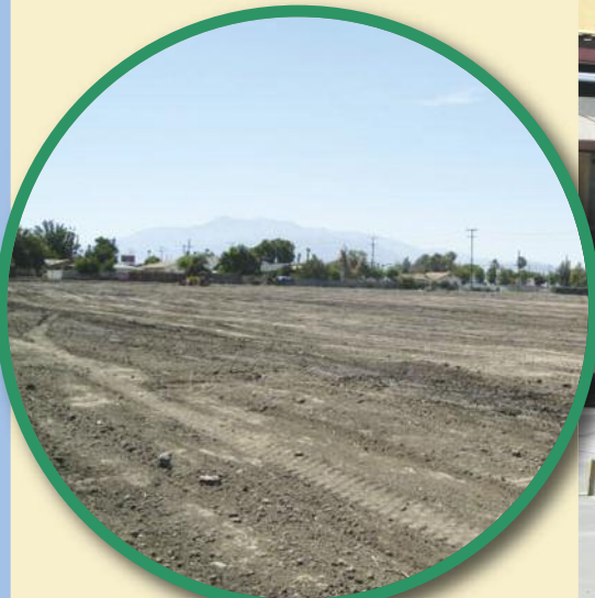
Graciano Gomez ES Site clearing completed
