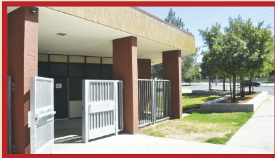
Emmerton ES Front entry to Administration Office remodeled
