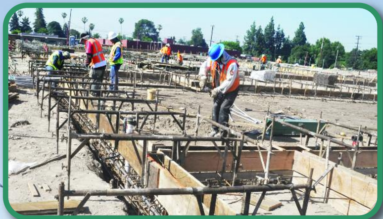
George Brown ES Administration Building footings
