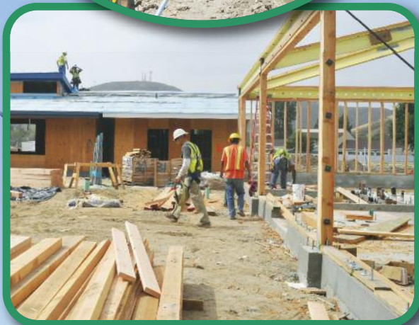
Little Mountain ES Multi-use Building erected
