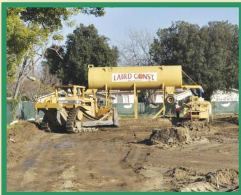
George Brown ES- Mass grading of the site
