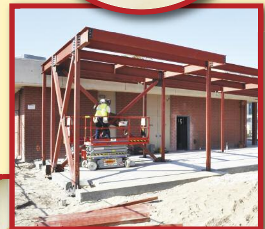
San Bernardino HS Steel Framing at Administration Addition
