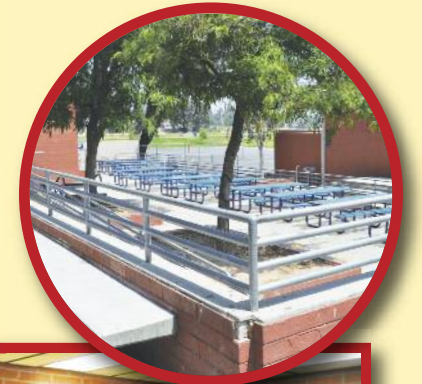
Serrano MS Shade Structure Area Before Demolition
