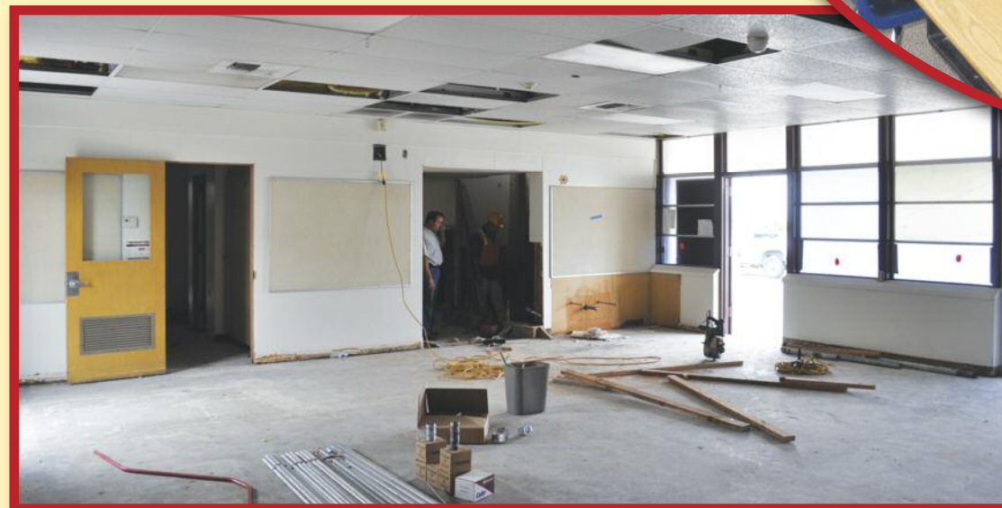
Cole ES- Kindergarten Classroom Under Construction
