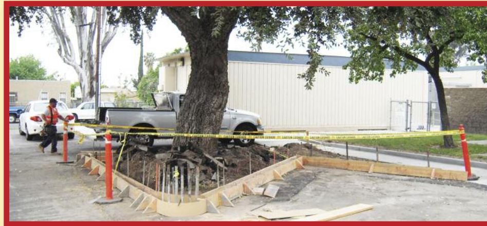
Burbank ES New Planter, Irrigation, and Curb installed at handicap Compliant Parking Lot
