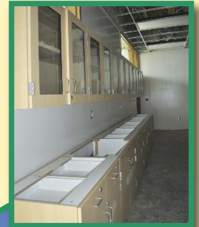
Indian Springs HS-Typical Science Classroom Under Construction
