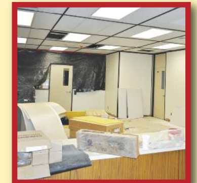
Richardson Prep-Removal of Ceiling and Floors are taking place at Administration Building
