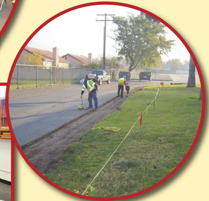
Lankershim ES New Fire Department Access Aisle and Irrigation
