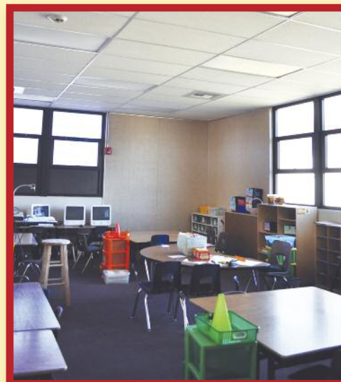
Bradley ES Typical Classroom Remodel: New Lights, Ceiling, HVAC Unit & Ductwork
