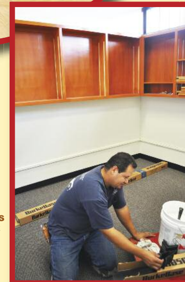
Highland Pacific ES Maintenance Work at Building E
