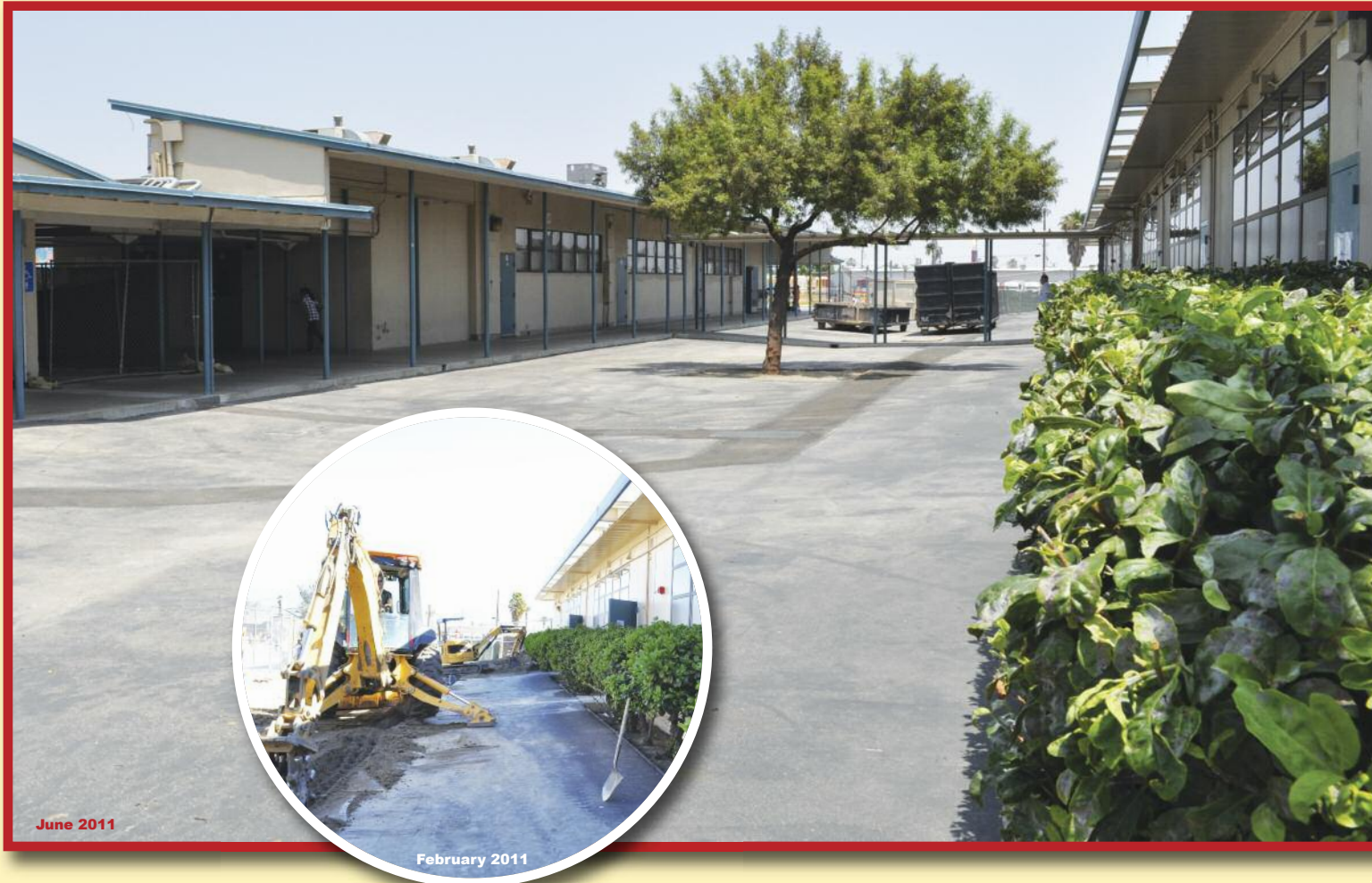
Lytle Creek- Underground Electrical and Data Feeding, Building E and Portables
