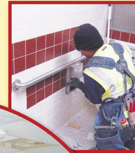
Lankershim ES-New Ceramic Tile and Fixtures at Remodeled Restroom
