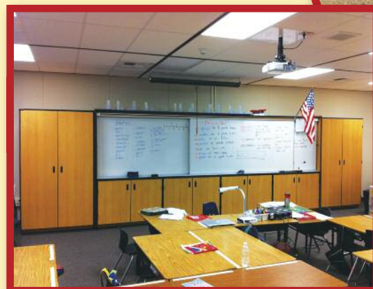
Lincoln ES Classroom Teaching Walls and Maintenance Work completed
