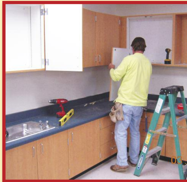
Burbank ES- A worker is installing New Cabinets and Sink in classroom
