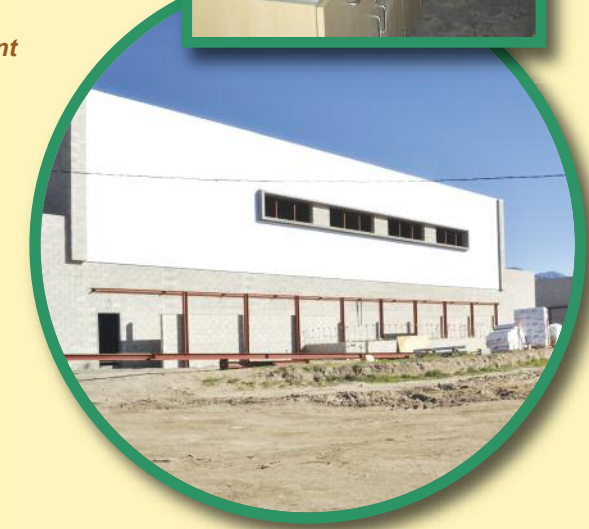
Indian Springs HS Building D Gym South Wall Fascia Under Construction
