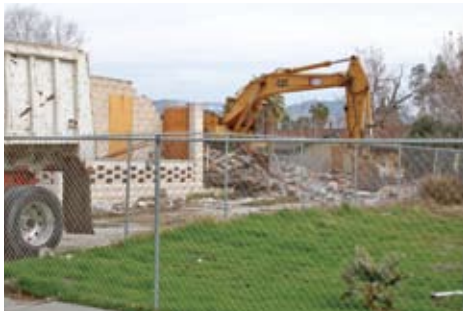
Demolition at the Norton ES site.
