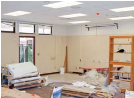
Cleanup efforts have started inside the teacher's lounge inside the Administration building at Hillside ES, where construction work has been completed.
