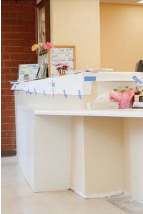
New casework installed at Carmack.
