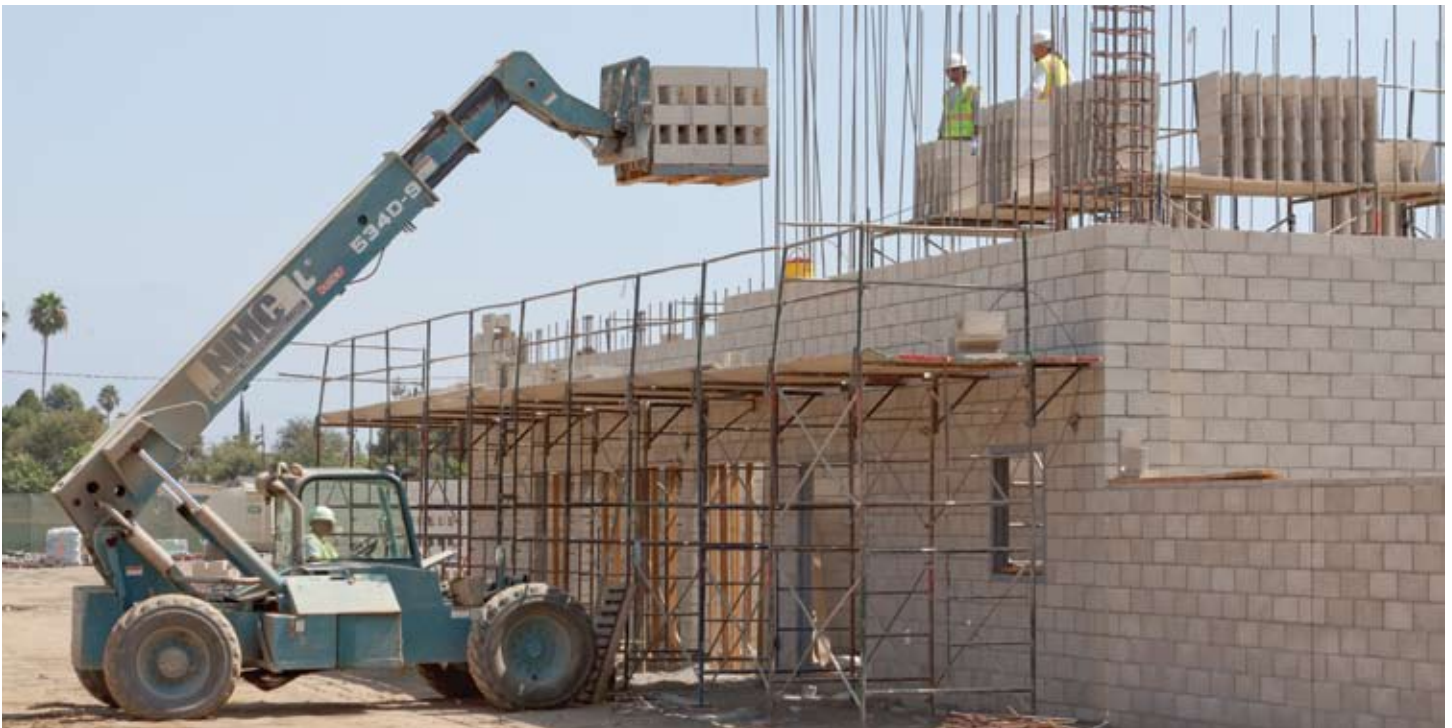
Workers continuing to do masonry work at one of the buildings.
