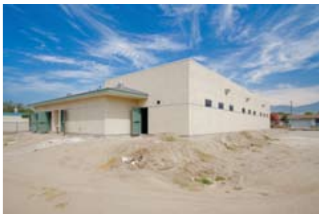
The SDC building as it was under construction at Rio Vista ES during 2009.
