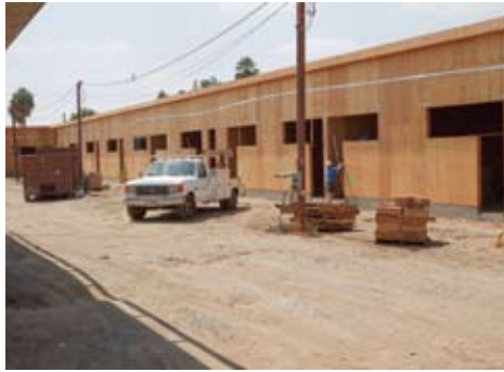
A row of new classrooms at Indian Springs HS.
