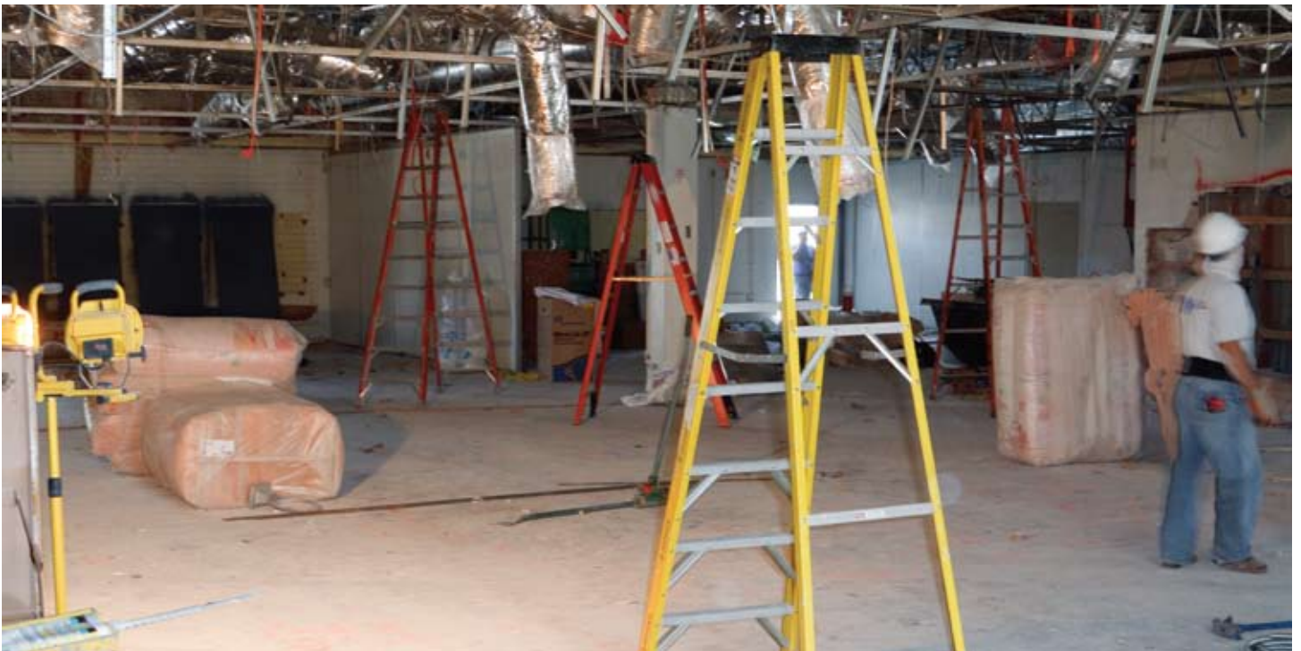
Installation of HVAC ductwork and insulation has started inside this building at Lincoln ES.
