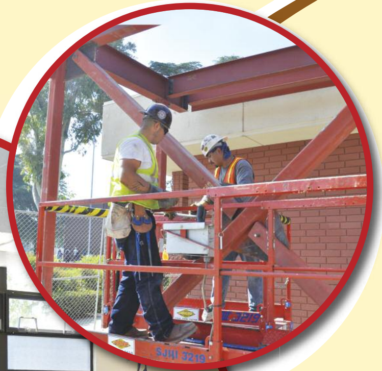
San Bernardino HS Steel framing at administration addition
