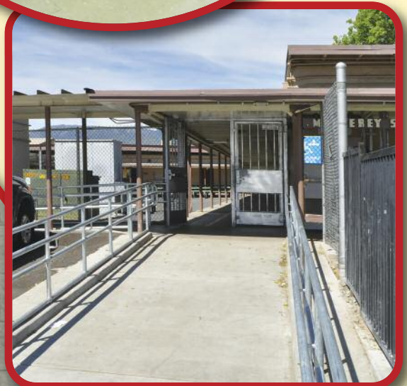
Monterey ES New ramp and path of travel
