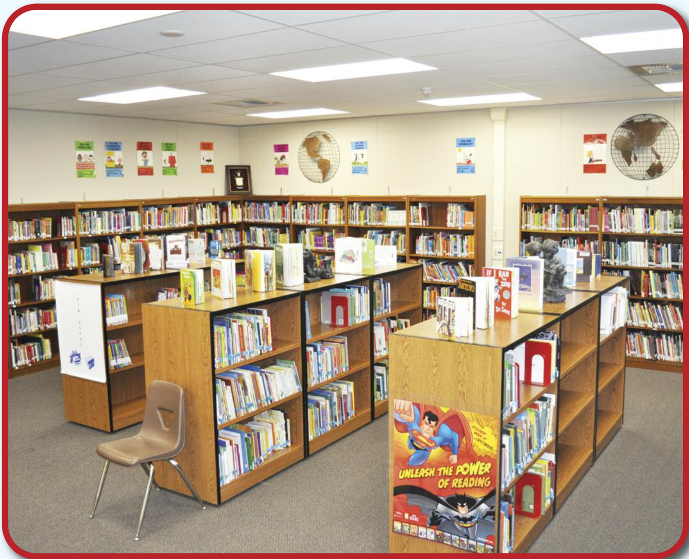
Hunt ES- Modernized library with new ceiling, lighting and flooring
