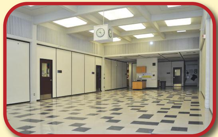
Riley ES- Modernized corridor with new flooring, partitions, doors, ceiling, lighting and paint
