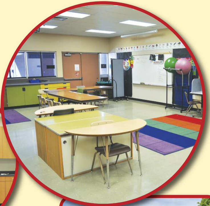
Anderson Special ED. Complete modernized classroom with new ceiling, lighting and flooring
