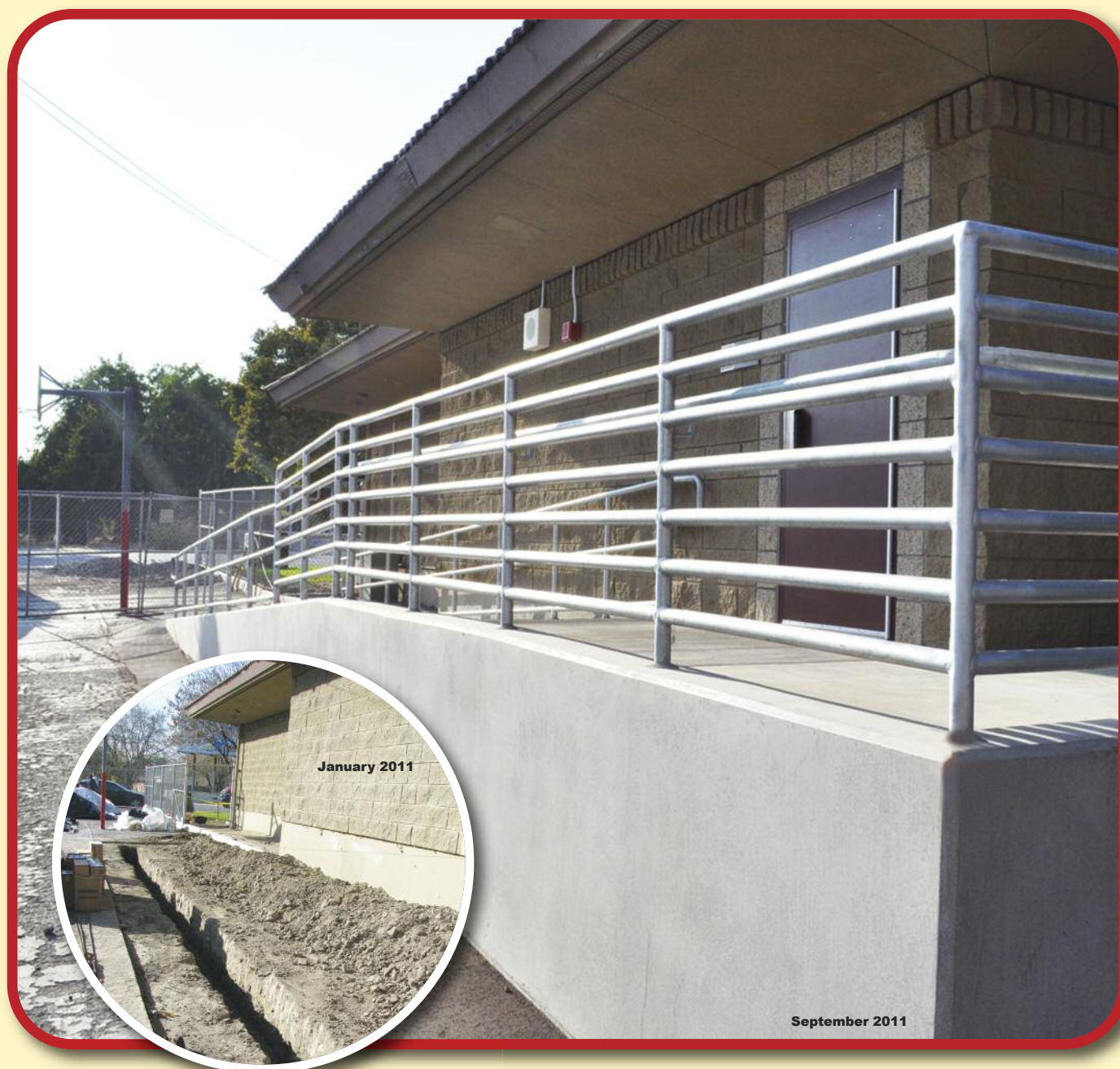
Mt. Vernon ES- New ramp at Building C under construction and finished
