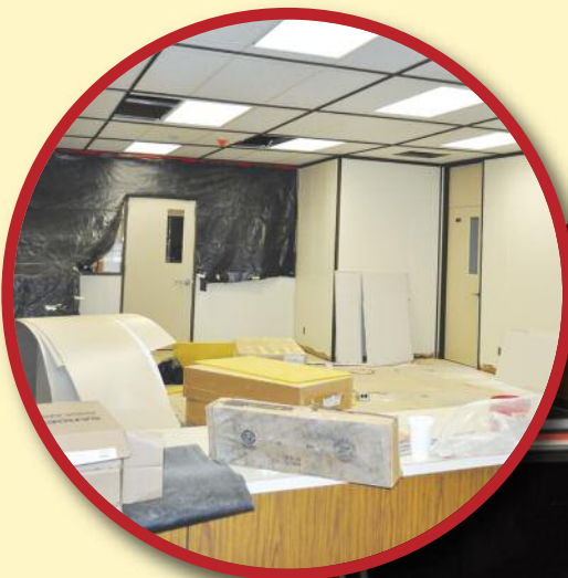
San Bernardino HS- Temporary administration office in Building B
