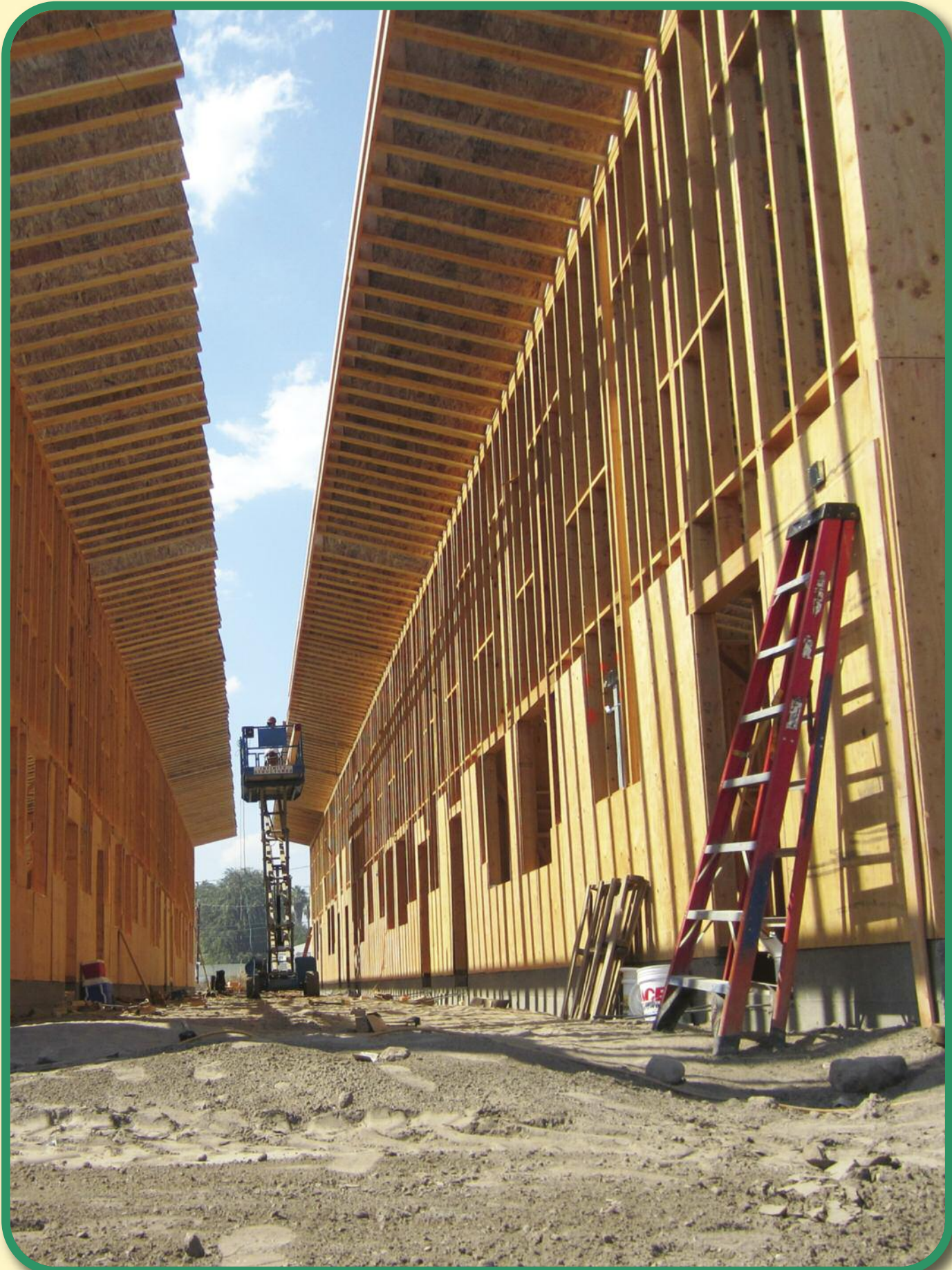
Captain Leland F. Norton ES- Building 6 framing under construction
