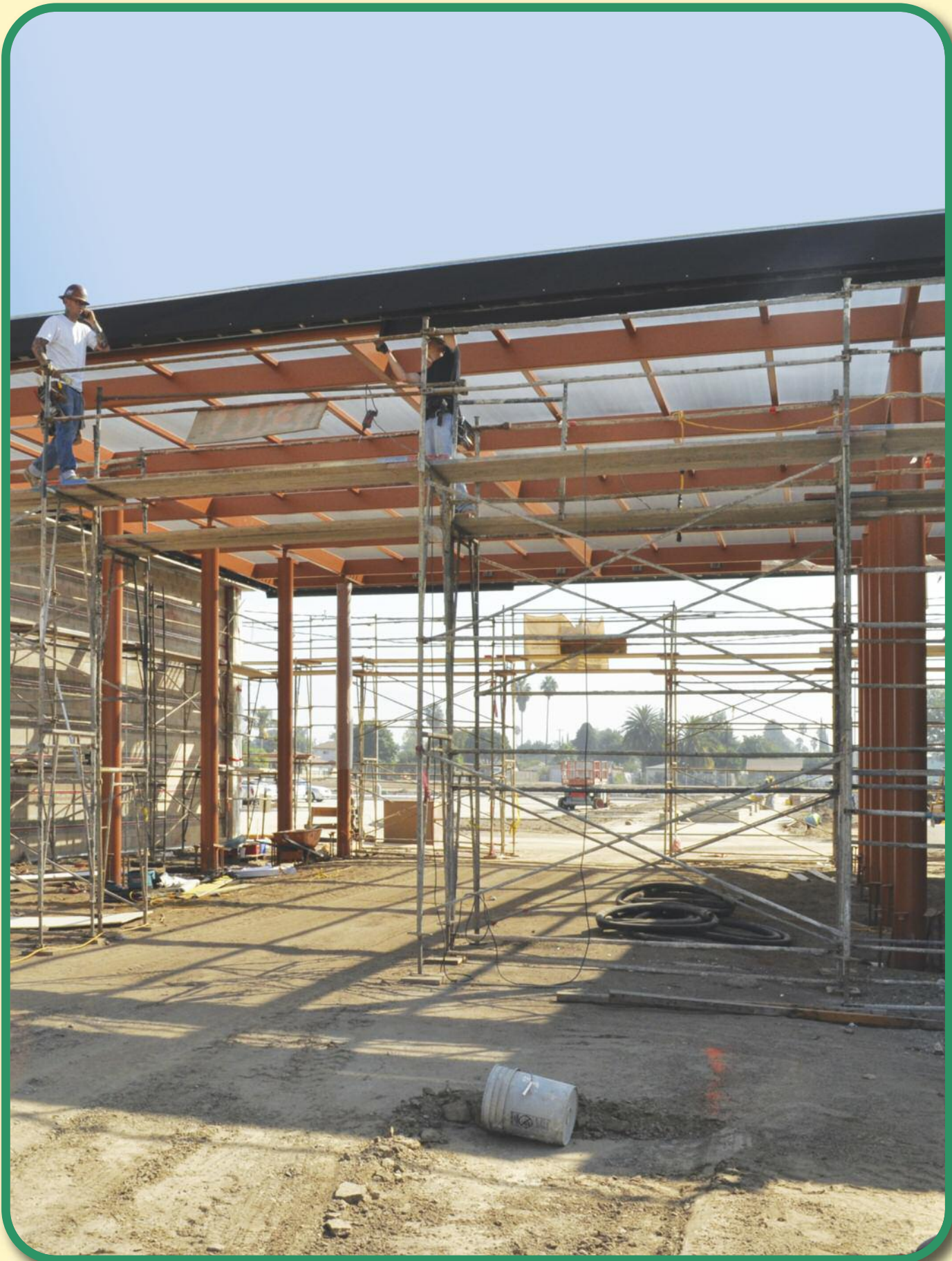
Indian Springs HS- Decorative steel trellis under construction at main entrance
