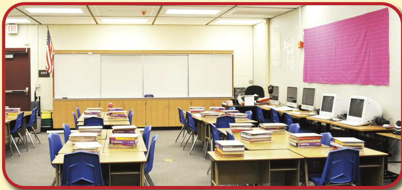
Ramona-Alessandro ES- Typical modernized classroom with new ceiling, lighting and teaching walls
