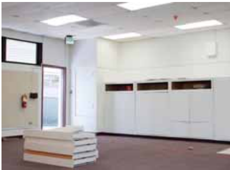
Recently remodeled classrooms at Cypress ES are having casework installed.
