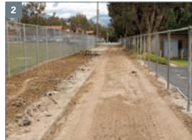
1 An old chain-linked fence has been removed and will be replaced with a new, safer fence. In the meantime, fence poles are being straightened before a new chain-linked “fabric” is installed. 2 Old asphalt has been removed from this utility road and will continue into parts of the playground. When completed, the new asphalt will redirect water for better drainage.
