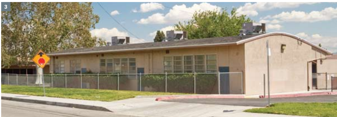
3 Buildings A, B (shown below), and C received new roofs to replace the existing ones.
