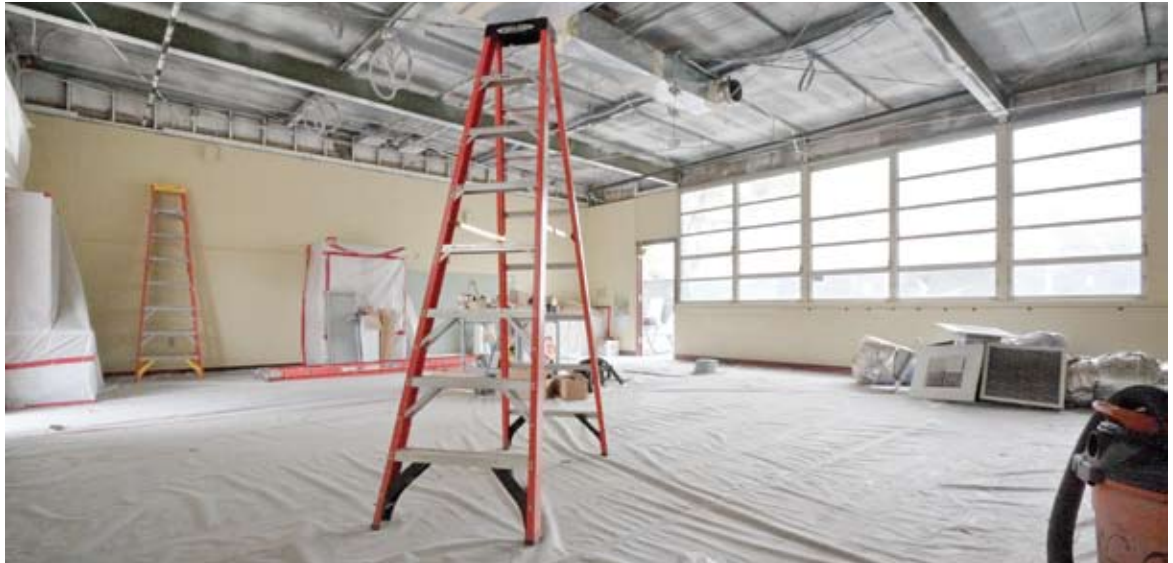
Modernization work has begun inside this Building B classroom, starting with abatement of existing materials.
