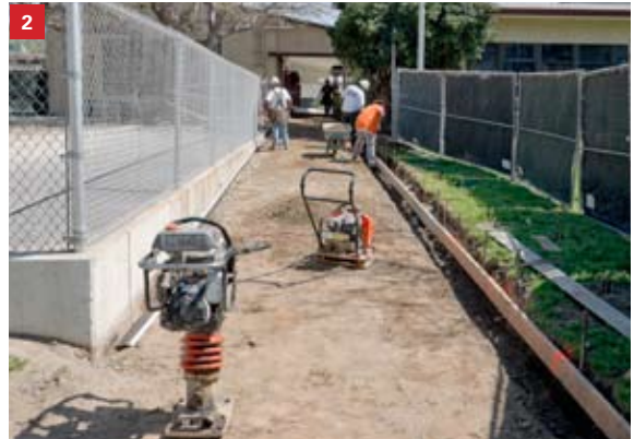
1 Portables have been fenced off at Hunt Elementary School as modernization work starts. 2 A new walkway leading to the front of the campus is under construction at Hillside Elementary School.
