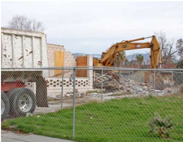
Top Location map for Norton ES. Above Site plan for Norton ES Left Some of the demolition that has taken place earlier this year.
