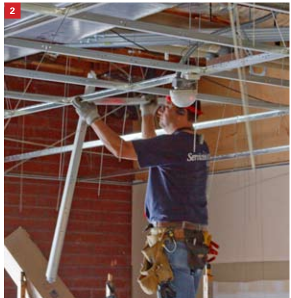
1 This restroom located between two classrooms inside Building D has been abated. 2 Installation of a new ceiling system inside one of two classrooms. Abatement work inside the classrooms and an adjacent restroom was recently completed.
