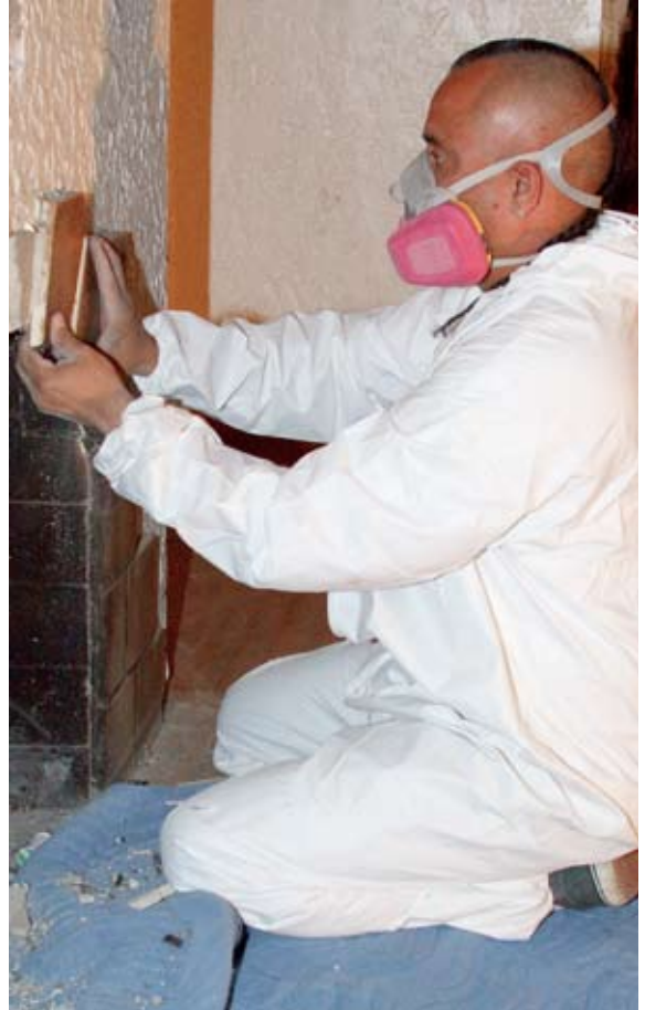
Right A tile carefully being removed from a fireplace. Some of the tiles will be saved and cleaned up for future use on the campus. Above and Below Details of some of the tiles on the fireplaces that were removed at the site.
