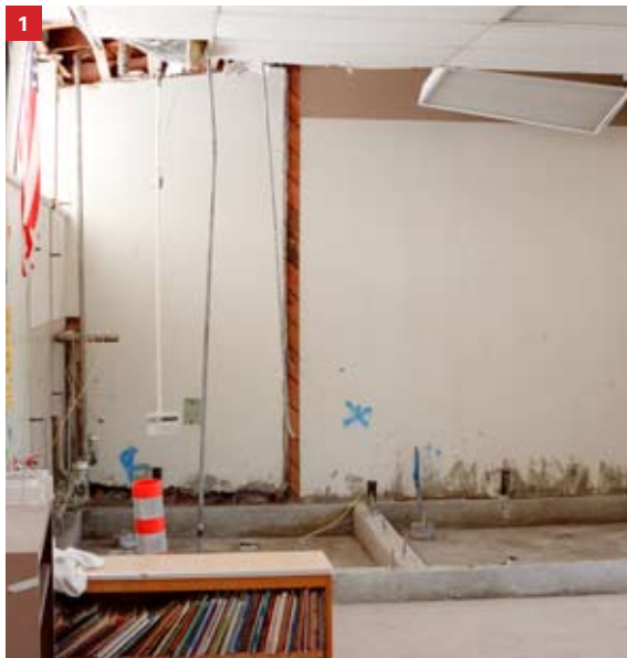
1 This restroom located between two classrooms inside Building D has been abated. 2 Installation of a new ceiling system inside one of two classrooms. Abatement work inside the classrooms and an adjacent restroom was recently completed.
