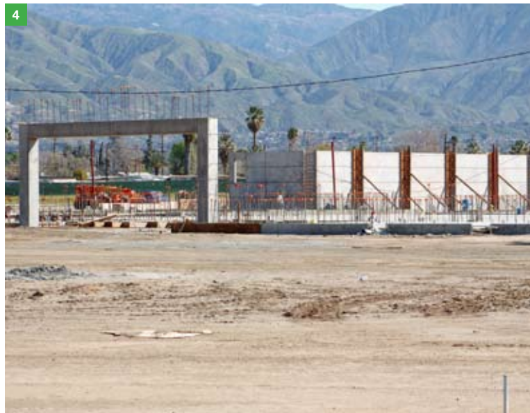
1 Stacks of lumber at the site that will be used in the construction of new buildings. 2 New wall framing continues to be built inside. HVAC work has also started. 3 A worker laying bricks that will be part of an extension wall at the future art labs. 4 Facades for both the gymnasium and locker rooms have been raised.
