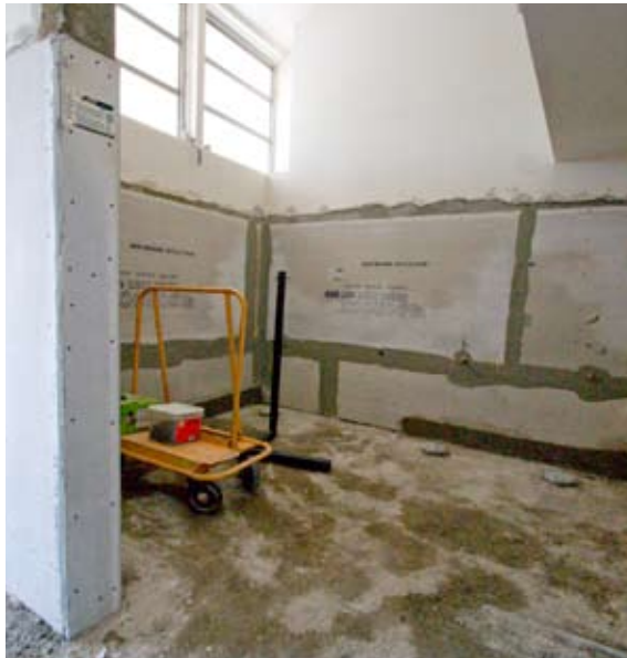
Left Inside one of the restrooms at Salinas where new drywall has been applied to the walls. Above Rough plumbing for an additional kindergarten restroom has been installed at Riley.
