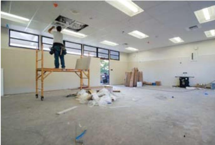
**Hillside ES** A worker installing a vent into the ceiling system of this classroom.
