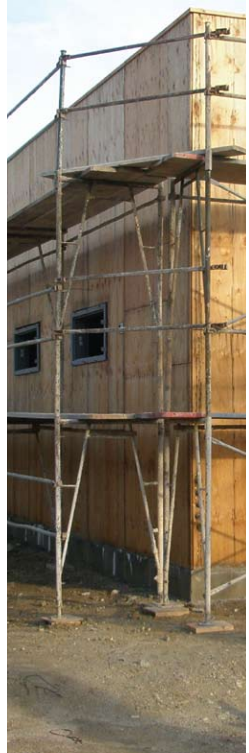
Hillside Elementary School SDC Building Work begins on the exterior stucco of the SDC building.
