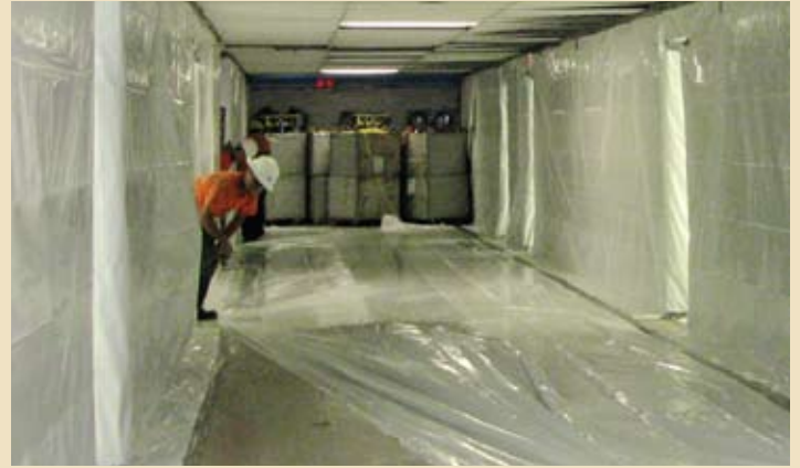
Workers begin to lay out protective covering on the walls and floors prior to working on the renovations.
