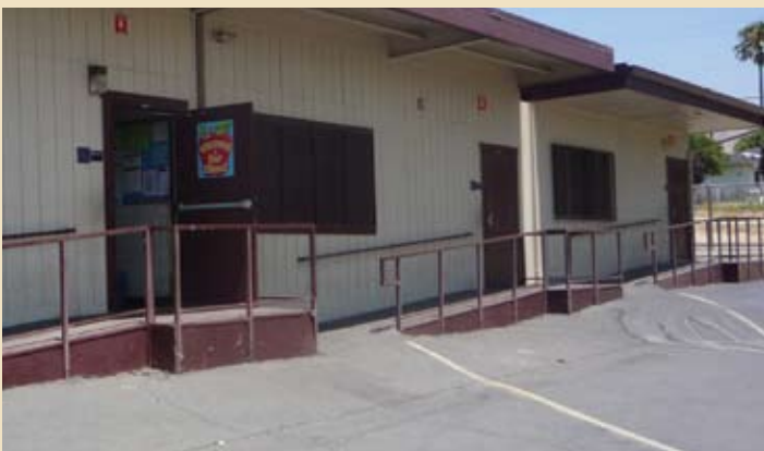
The project includes updating existing ramps to make them more ADA compliant, including these found at Hillside Elementary School.
