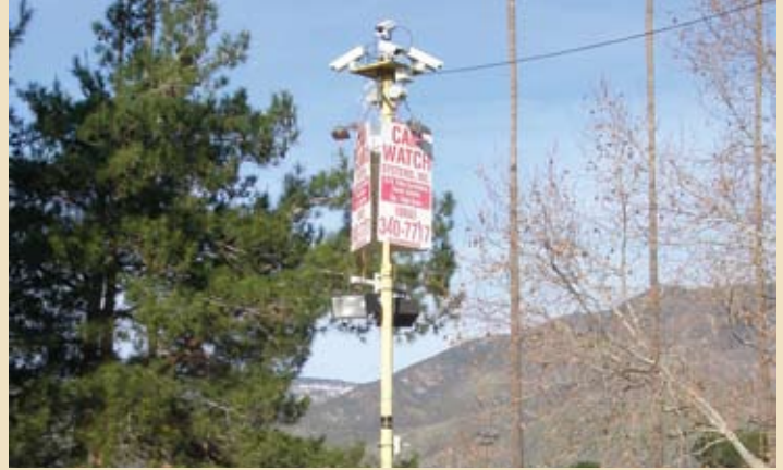
Temporary monitored security camera system and temporary power connection for construction have been installed.
