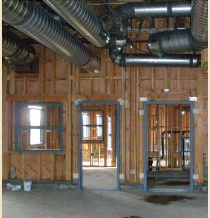
Frames for doors and windows have been installed. Rough-in work has also been completed for HVAC duct work and electrical conduit.
