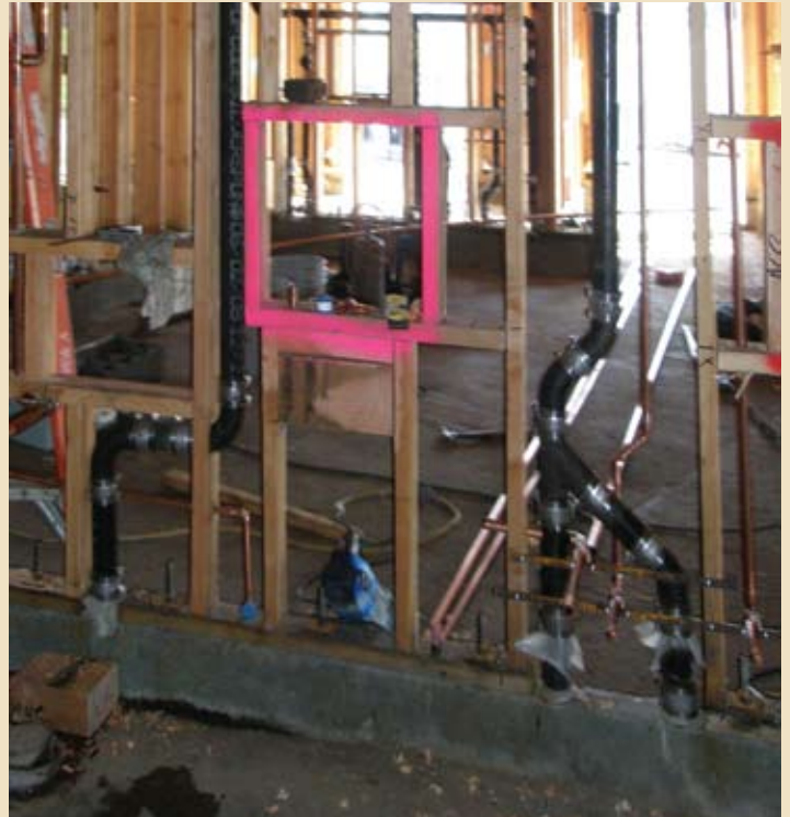
Inside, progress continues as rough-in plumbing to the building has been installed.
