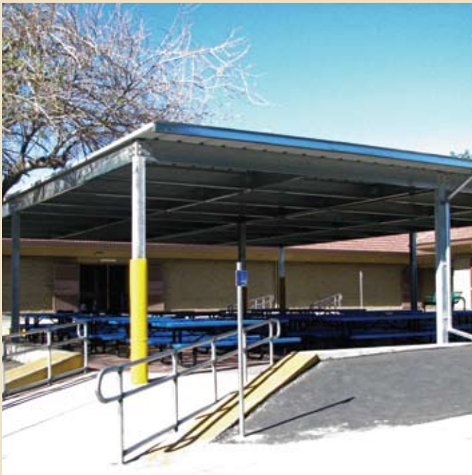
Mt. Vernon Elementary School lunch shelter protects students from the sun and rain.
