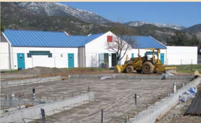
With stem walls complete and underground utilities trenched and back-filled, rebar and concrete slab will be installed next.
