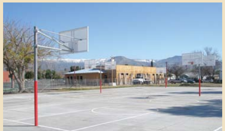
As part of the project, a new concrete basketball court was built to replace the old court where the SDC building now stands.
