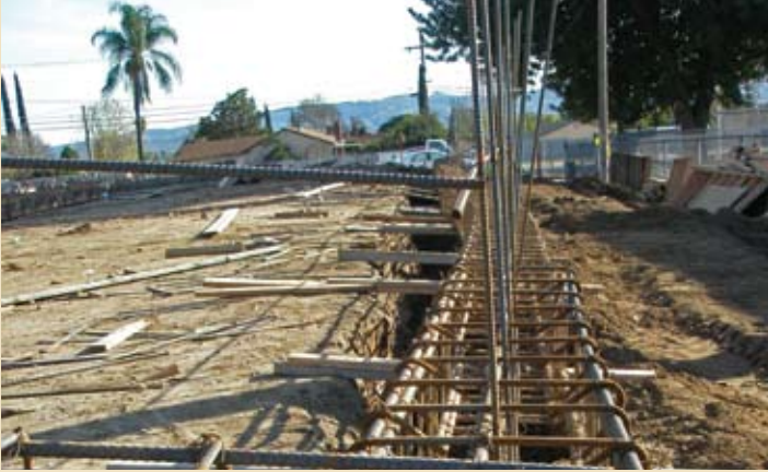
Grade beams and stem wall rebar/form work for the concrete pour are finished.
