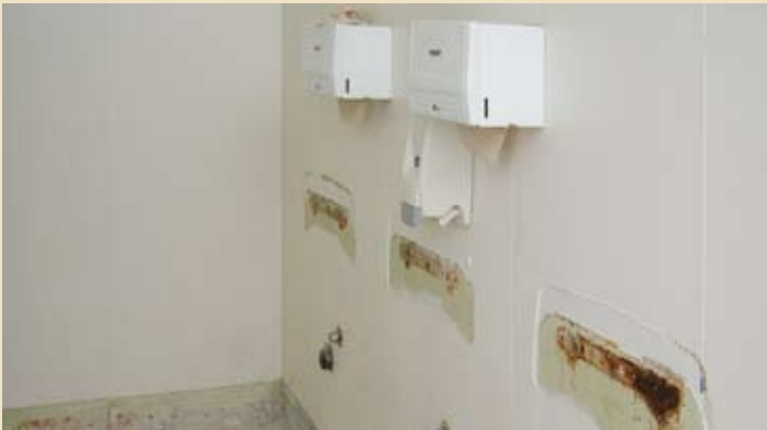
A restroom at Fairfax Elementary School, where existing sinks and fixtures have been removed are being prepped for modernization.
