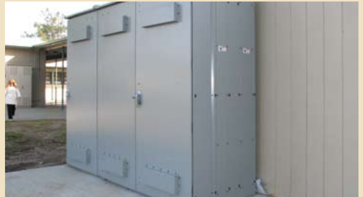
New electrical panels, including this one at Warm Springs Elementary School, are being installed in anticipation of modernization work that includes electrical wiring upgrades throughout the campus.
