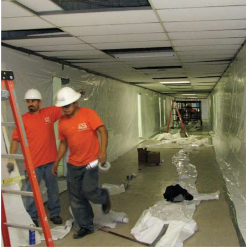
San Geronio High School Modernization Workers prepping the school for renovations.
