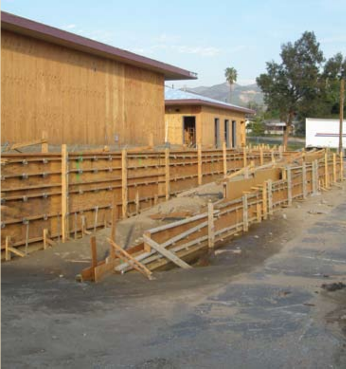
Form work for a retaining wall and ADA-compliant ramp have been built.
