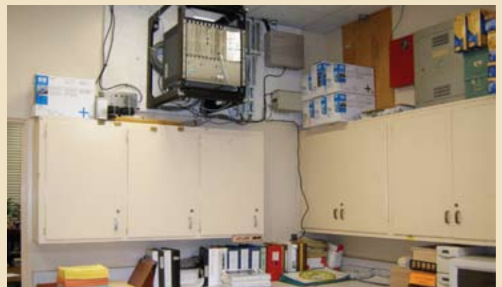
Hunt Elementary School will receive upgrades, including electrical, data, security, and energy management systems.
