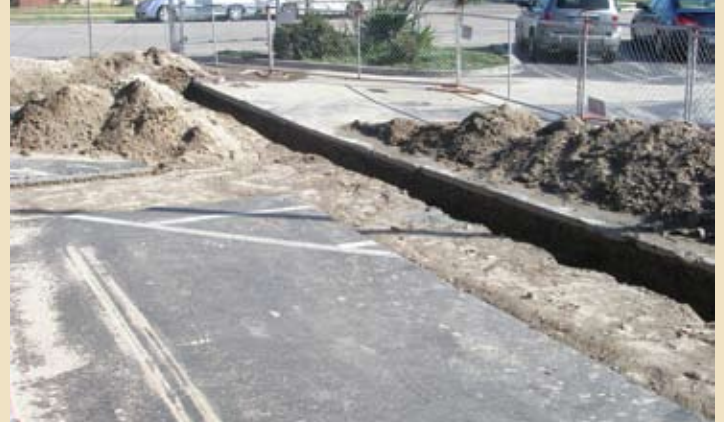
Outside, trench work has been done to install utilities into the building.
