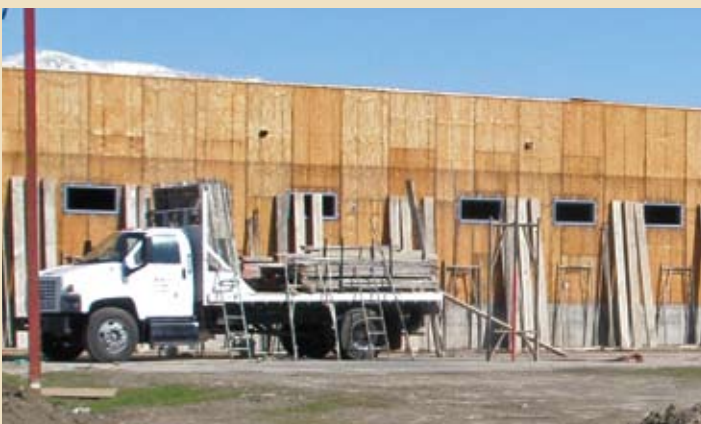
Scaffolding is being erected to commence work on the exterior stucco.
