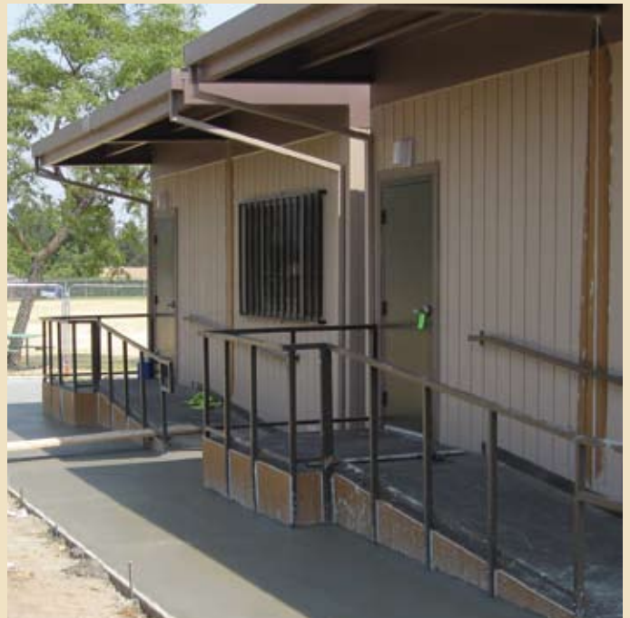
This QEIA project consisted of design, sitework, and installation of 29 portables classrooms at 10 sites.
