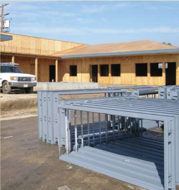
Metal door and window frames sit outside of the site and will be installed in the coming days.
