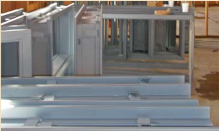
Metal door and window frames have arrived to the site.
