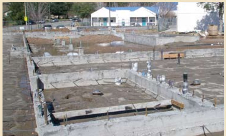
Stem wall rebar will be tied into concrete slab rebar that will be placed next.
