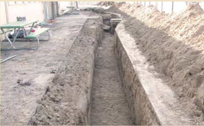
Trenching for remote utility connections have been dug.
