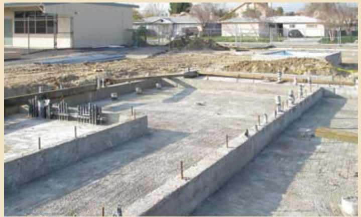
Stem walls and slab-on-grade have been poured. The wall framing and anchor bolt connections are starting to be built.
