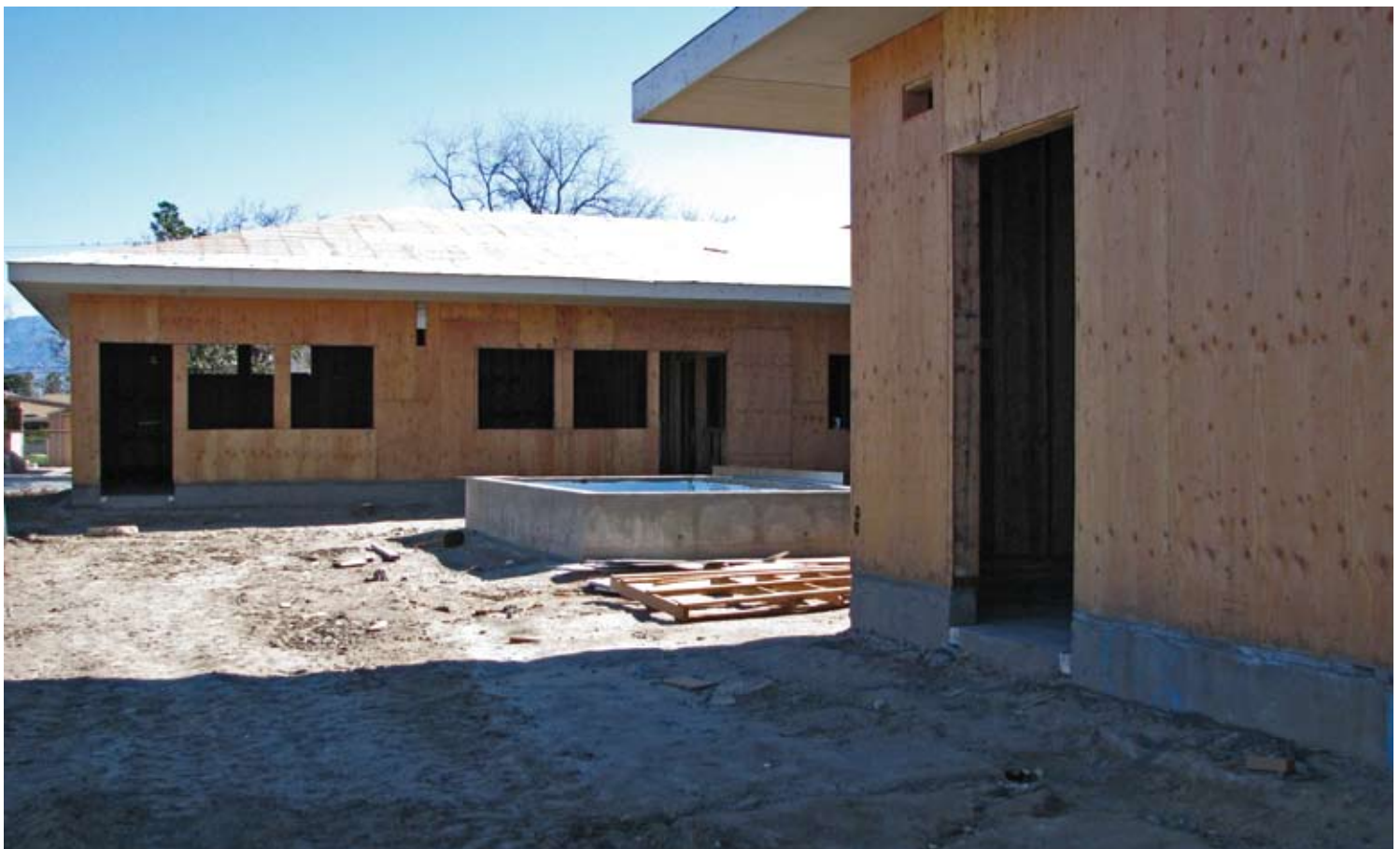
Bradley Elementary School SDC Building Side and courtyard view. When completed, the planter inside the courtyard will allow students to learn about growing and maintaining food and plants.
