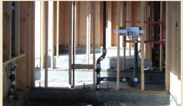
Rough-in plumbing work has been installed.
