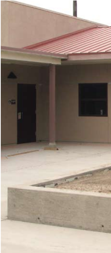
Highland-Pacific ES This SDC building, along with the remaining buildings, are nearing completion.
