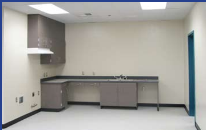
This kitchen area is waiting for appliance delivery and installation.
