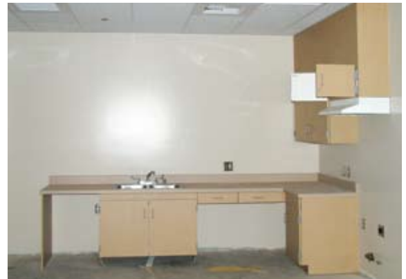
Casework installation for all of the classrooms has been completed. Carpets and tiles are to be installed next.
