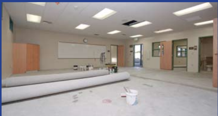
Carpet and tile installation continues inside the classrooms, restrooms, and offices.
