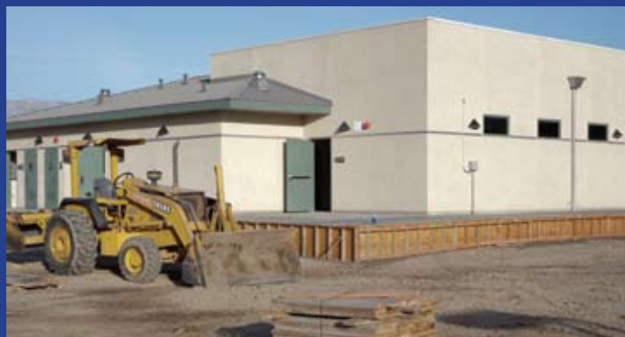
Outside, concrete walkways have been poured around the building and the area is being prepped for asphalt.
