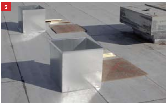
Building E has recently been completed and classes have resumed, including this art class (1) and the newly completed band room (2). 3 Modernization work has started in Building B. A bulldozer is removing what was once a stage. 4 This restroom has been completed gutted. Rough plumbing work is currently being performed inside. 5 On the roof, holes are being cut to install the skylights throughout. 6 In another part of Building B, special exhaust fans filter air out of the building.
