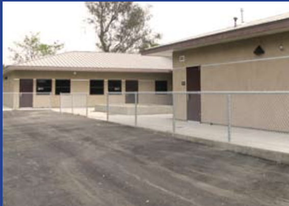
New fencing is installed and asphalt poured around the perimeter of the building.
