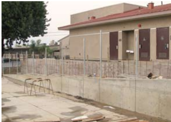
A new ramp and railing system is under construction that will allow easy access to the new building.
