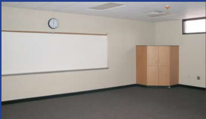
With casework and flooring now complete, efforts are now being concentrated on final preparations.
