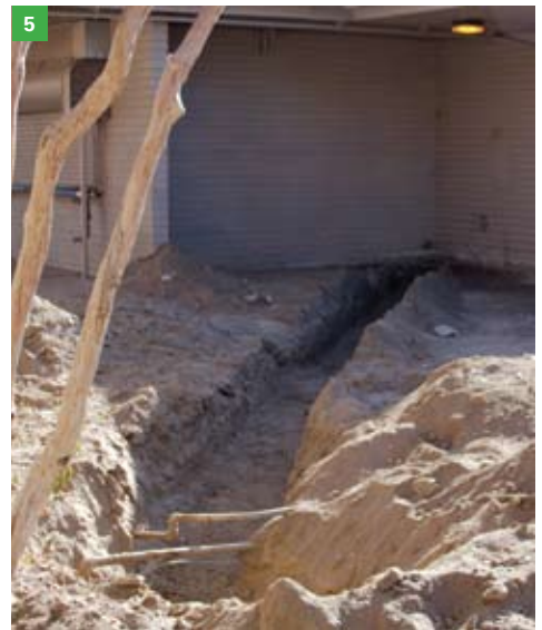
1 The inside of Building A has been completely abated, leaving only the exterior walls. 2 This headwall installed at the northern portion of the site will provide drainage throughout the campus and prevent erosion. 3 A dump truck being loaded with debris from Building A. 4 Electrical utility boxes waiting to be installed. 5 A trench for rough plumbing dug near the existing cafeteria.
