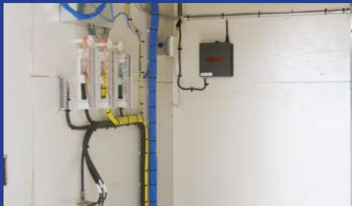
The building has been wired for data and voice lines. Other systems, such as emergency alarms, have also been installed.
