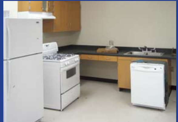
With the new flooring put in, final tasks such as appliance installation are now taking place.
