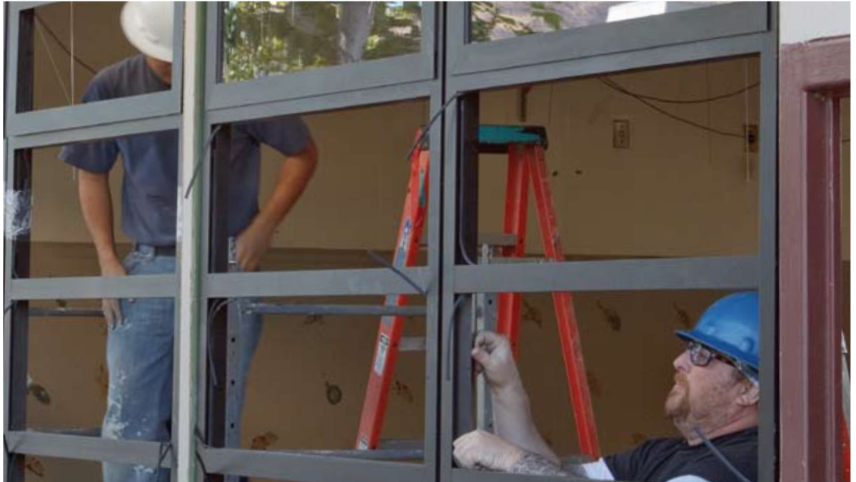
Hillside ES Workers installing new windows inside a classroom in Building F.
