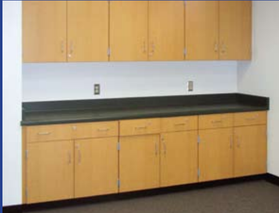
Casework and flooring have been installed throughout all of the classrooms and offices.
