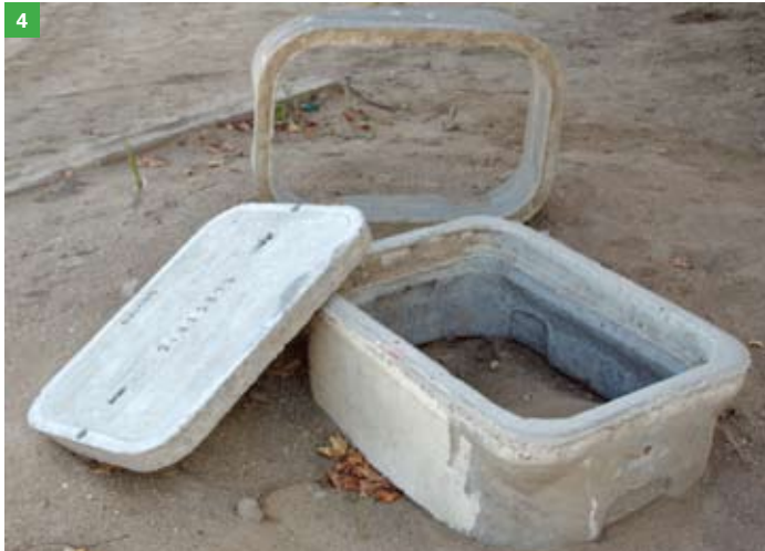
1 The inside of Building A has been completely abated, leaving only the exterior walls. 2 This headwall installed at the northern portion of the site will provide drainage throughout the campus and prevent erosion. 3 A dump truck being loaded with debris from Building A. 4 Electrical utility boxes waiting to be installed. 5 A trench for rough plumbing dug near the existing cafeteria.
