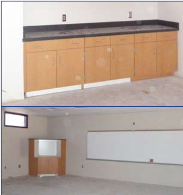
Casework in the pullout room (top) and in a classroom is complete.
