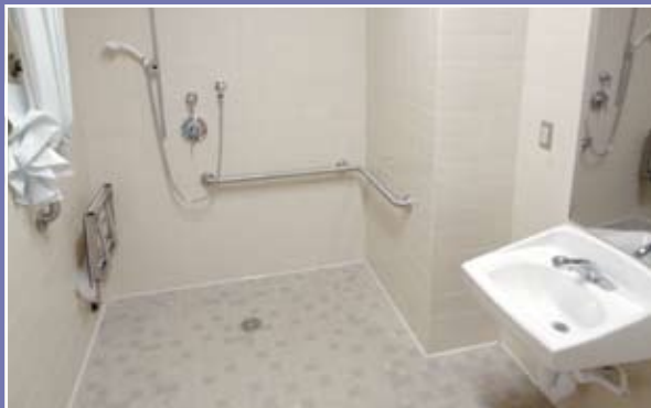
A typical restroom inside the SDC building, featuring shower facilities.
