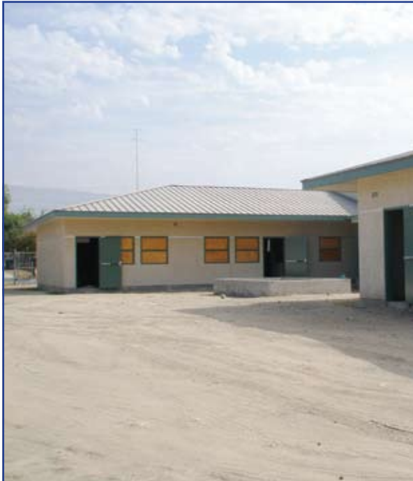
The area surrounding the building has been graded for concrete and asphalt installation.
