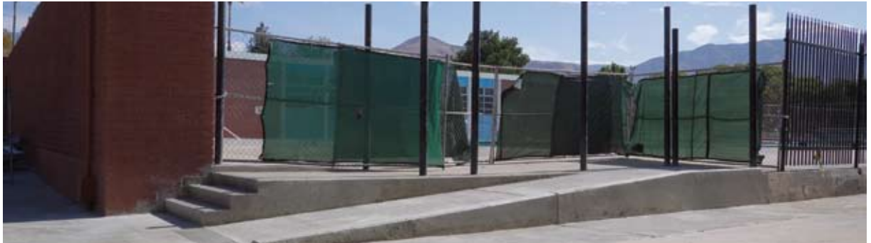
Construction of upgraded stairs and a new ADA-compliant ramp are completed at the swimming facilities. New fencing and handrails will complete this portion of the project.
