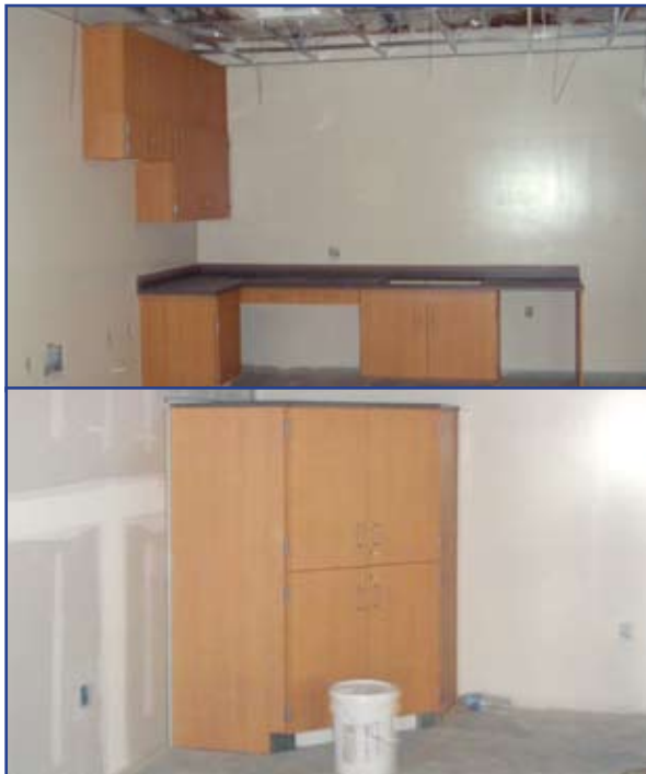
Casework installation begins. Shown are cabinets for (top) a typical kitchen area and (bottom) video equipment storage.
