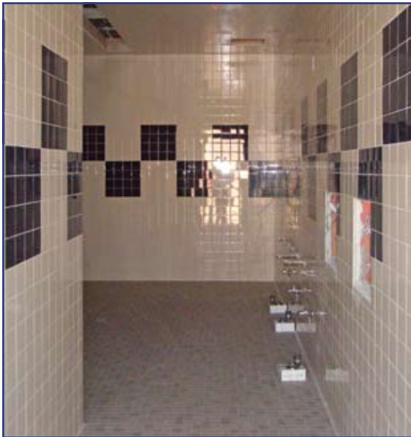
Tiles have been set on the walls and floors in the restrooms. Sinks, hand dryers, and other finish work will begin shortly.
