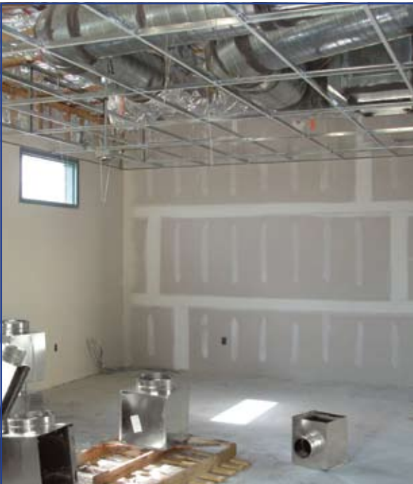
Finish ventilation and ductwork installation continues inside.
