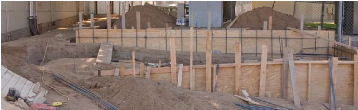
Hillside ES A new ADA-compliant ramp being constructed near the front entrance of the school.
