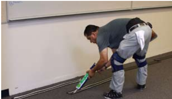
A worker installing rubber baseboards around a classroom in Building C. Carpet and tile installation progresses as well throughout the building.
