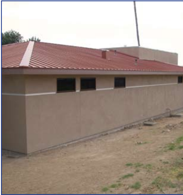
Installation of utility boxes outside the building. All utilities are now connected with the main campus.
