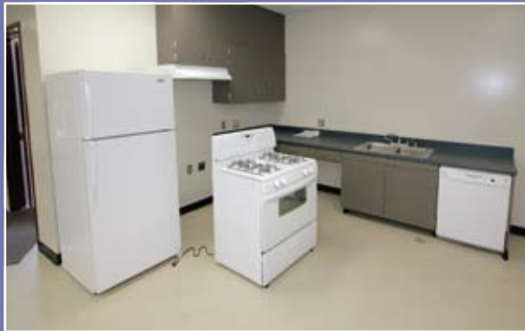
Typical kitchen facilities. All of the appliances being installed are energy efficient.
