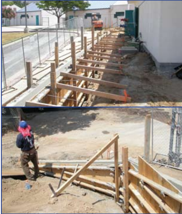
Workers frame future ramps and retaining walls that surround the building.
