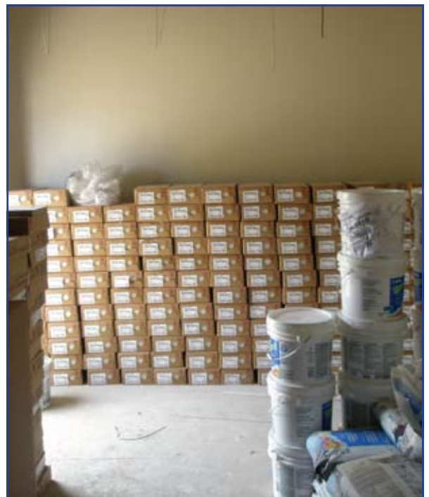
Boxes of tiles and tubs of plaster that will be used for floor installation.
