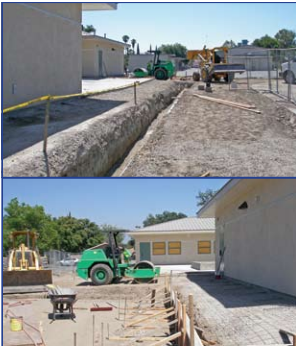
Rebar and formwork is in place for the concrete walls and walkways to be poured.
