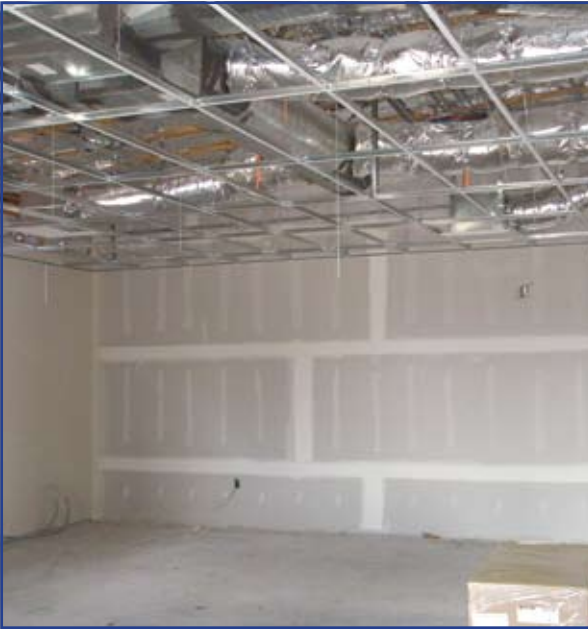
Sheetrock installation is complete. Framework for ceiling tiles are also in place.
