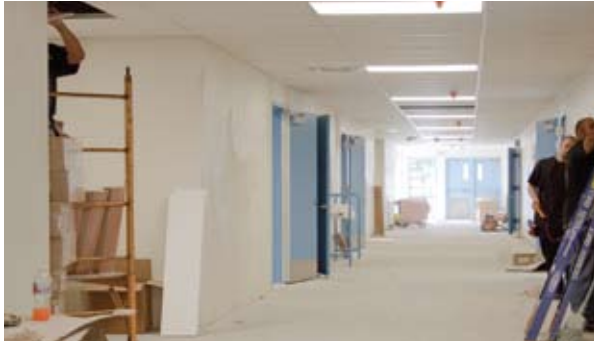
Inside Building C, lighting and ceiling panels are being installed. The interior walls have been given a fresh coat of paint. New public address and fire alarm systems were upgraded as well.
