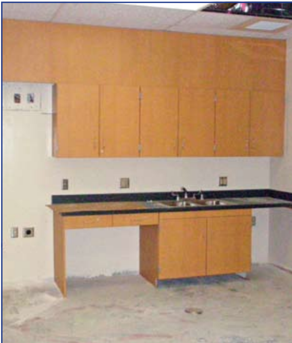
Casework installed in the kitchen. Tiling and carpets will be installed afterwards.
