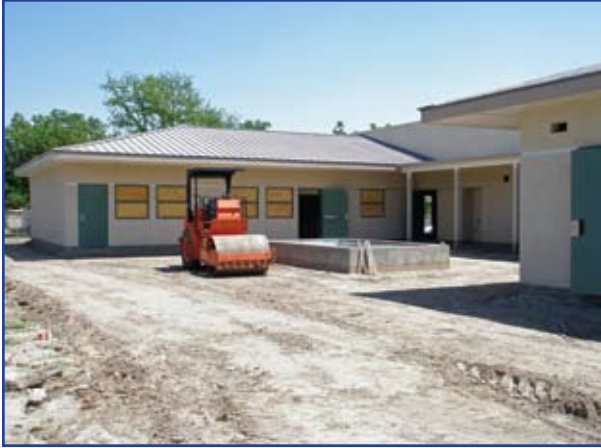
The grounds outside the building are prepared for cement walkways and landscaping.
