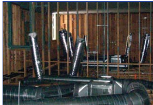
Duct work for heating & ventilation are being prepared for installation.
