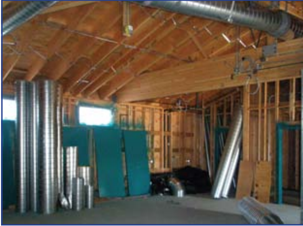
HVAC ducting and steel doors and jambs delivered; installation has started.
