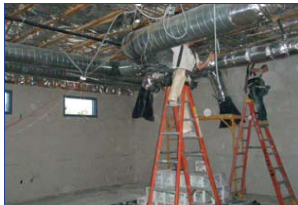
Inside, workers pull electrical wire throughout the building. Sheetrock and insulation have been laid on the walls.
