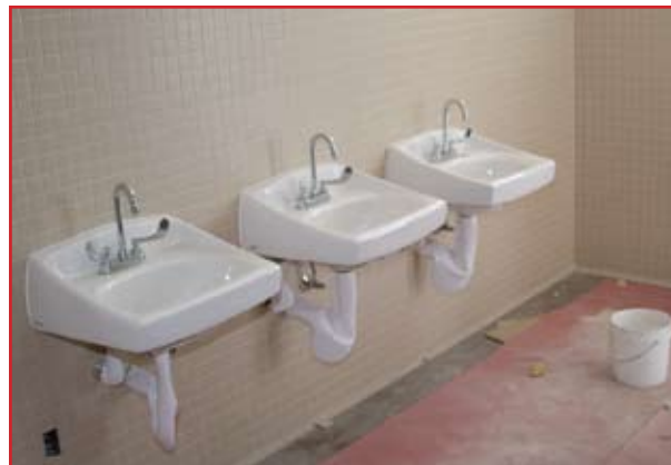
Warm Springs ES Renovated restrooms featuring ADA-compliant fixtures for easier accessibility.
