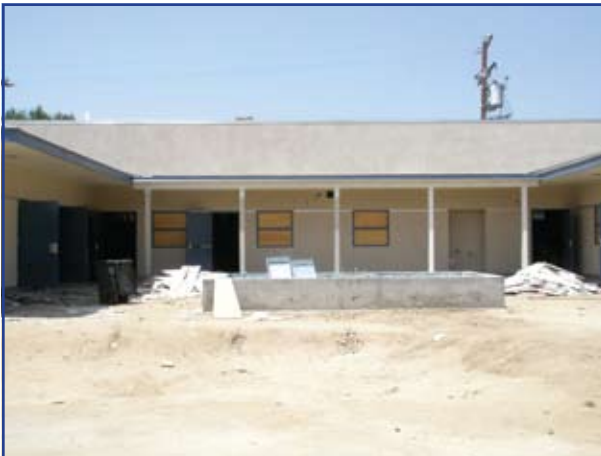
With the building exterior nearly complete, the next phase will be to install walkways and landscaping.
