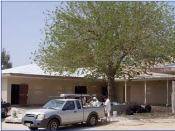
Workers apply the final layer of paint to the exterior of the new building.
