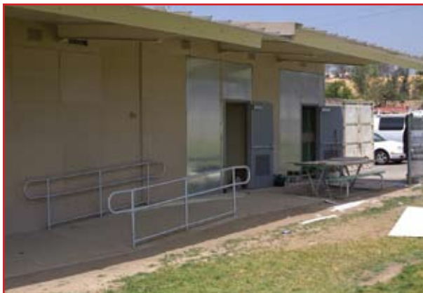
Fairfax ES A new ADA-compliant ramp leads to renovated restrooms.
