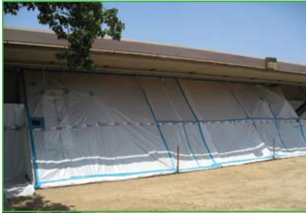
Hazardous materials are abated from the inside of existing buildings.
