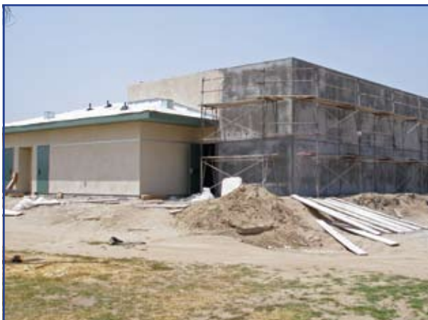
The final color coat is being applied to the stucco of the building.
