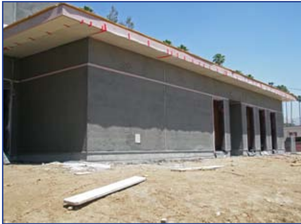
The third "scratch" coat has been applied to the exterior of the building.
