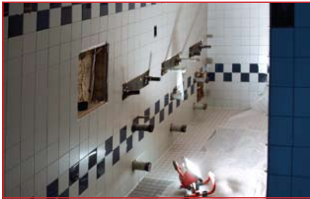
The new restroom facilities will include new fixtures and ADA-compliance upgrades.
