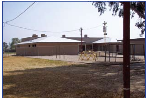
When complete, the new SDC building will contain 3 classrooms, a kitchen, a laundry room, and offices for staff.
