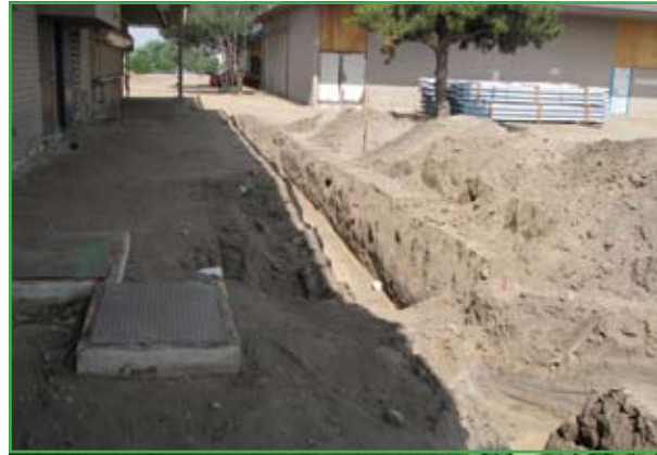
Trenchwork for sewer, water, and electrical lines are dug inside the courtyard areas.
