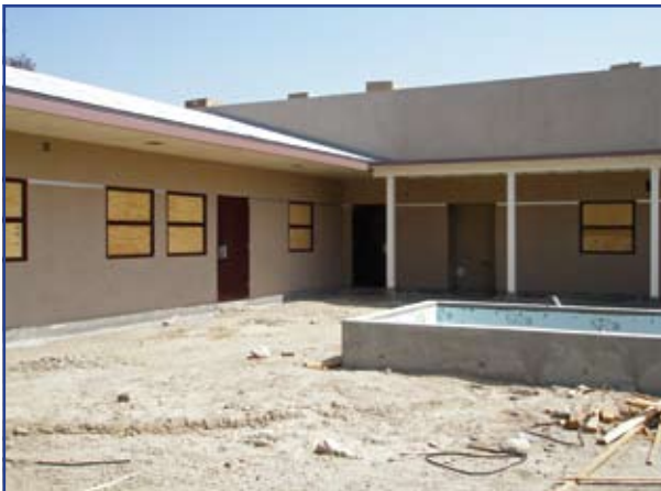
Steel window frames and doors installed. The exterior was also given a fresh coat of paint to complete the stucco process.
