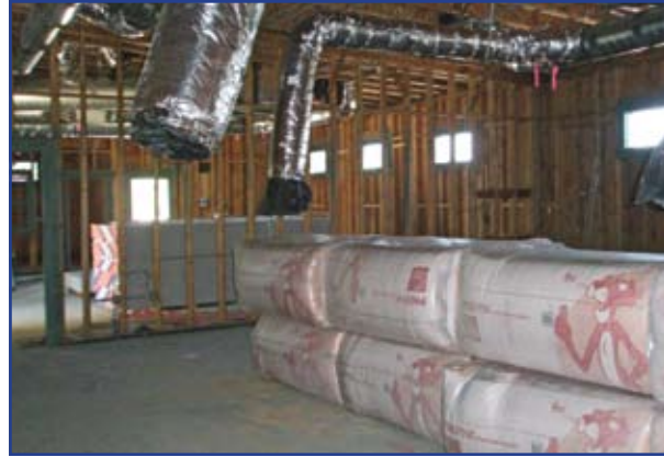
Sheetrock and insulation delivered and pending installation.
