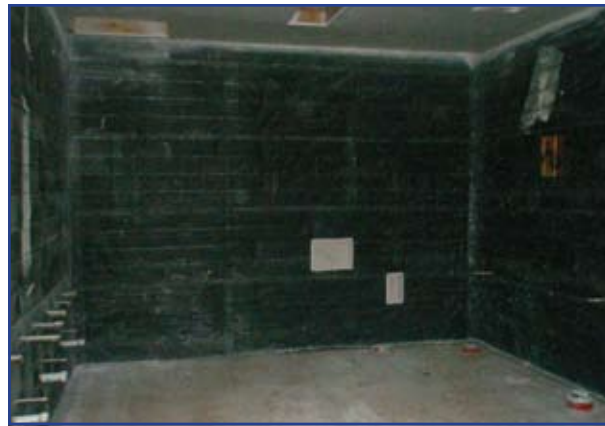
The walls of the restrooms are covered in paper in preparation of tile work.
