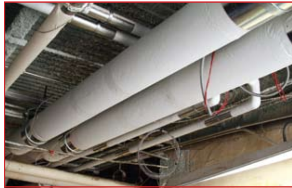
Special hydronic pipes installed in the ceiling are used in heating and air conditioning applications.
