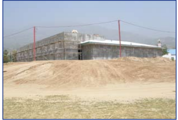
The stucco layer has been applied and is currently drying prior to the final color coat.
