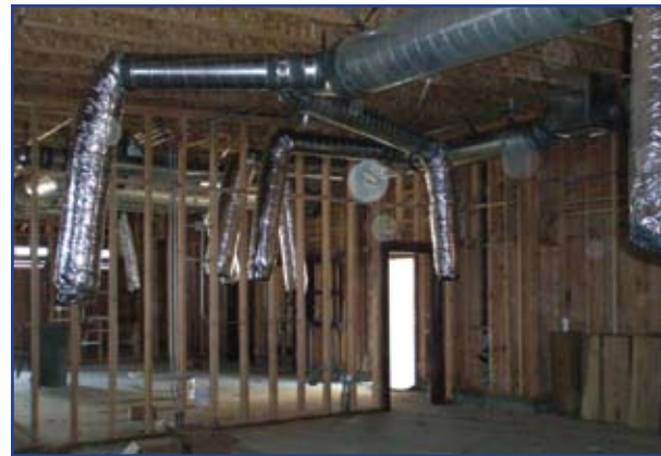
The beginning stages of HVAC duct work have been installed.
