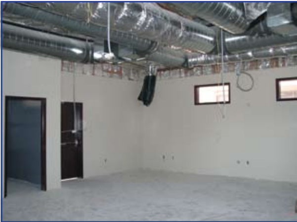
Insulation and sheetrock are now on the walls. Electrical conduits also installed in preparation of final electrical work.
