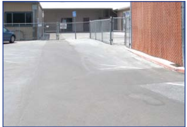
All the trenchwork completed previously is now filled in and asphalt laid on top.
