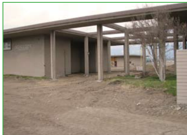
Existing former Curtis Middle School building exterior courtyards have been demolished; interiors have been deconstructed for modernization.
