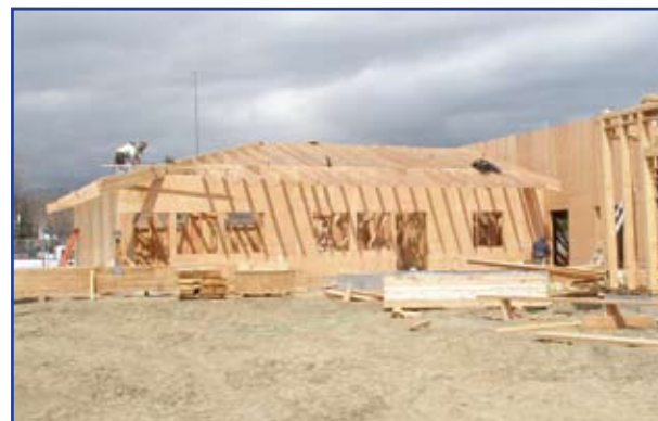
Initial phase of rough framing with enclosure of exterior walls and roof are underway.
