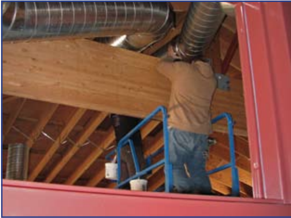
Tradesmen work on HVAC system ductwork.
