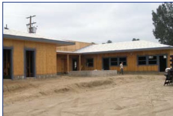
Rough exterior sheathing is complete; water resistant membrane tacked in place on roof protects ongoing interior utility work and materials.
