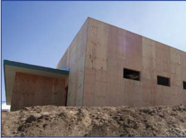
13,000 cubic yards of clean fill elevate this building to at-grade of existing campus.
