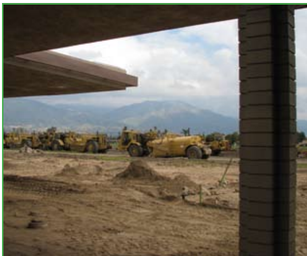
Sitework at the former Curtis Middle School includes grading and utility trenching of adjacent newly acquired 43 acres.
