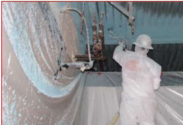
A worker sprays chemical flame retardant in Building C; electrical upgrades to follow.
