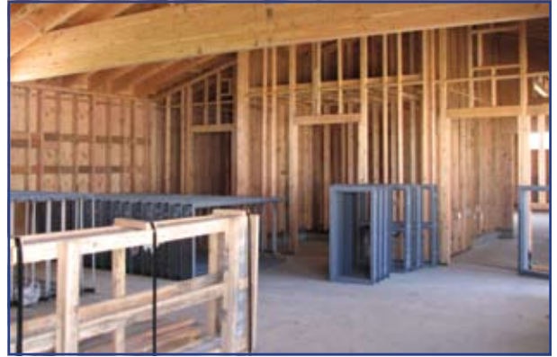
Metal door and window frames delivered for installation.
