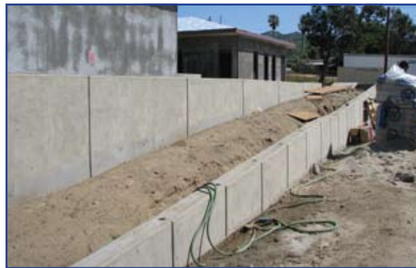
Concrete retaining walls for ADA-compliant ramp cured; the fourth layer or "brown" coat of plaster is curing on building exterior prior to final 5th layer or "color" coat.
