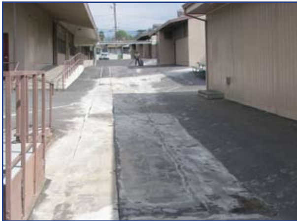
Plumbing remote lines began with saw cutting of asphalt while school is off-track to minimize classroom disruption.
