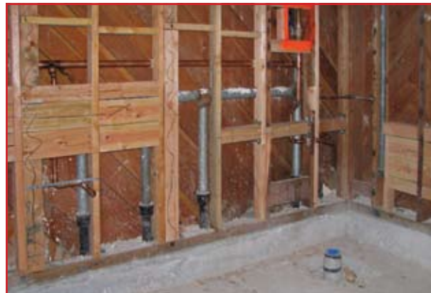
Warm Springs ES Modernization scope includes complete plumbing remodels.
