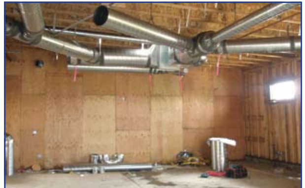
HVAC ductwork is being installed.
