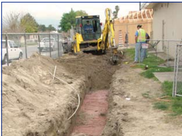
Trench work along side of school is for utilities that will tie-in to existing system.
