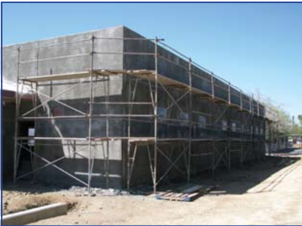
The third, or "scratch", plaster coat of the 5-layer stucco process applied.
