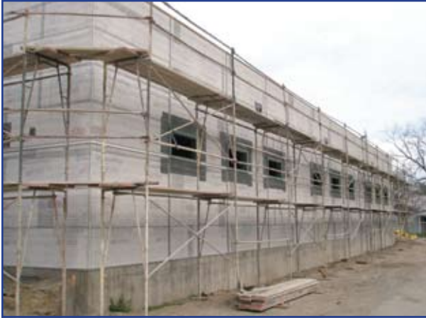
In place are water resistant membrane and metal lath which are the first 2 layers of a 5-layer plaster and stucco process.
