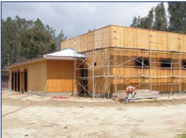
The assembly of scaffolding signals the start of exterior stucco work.
