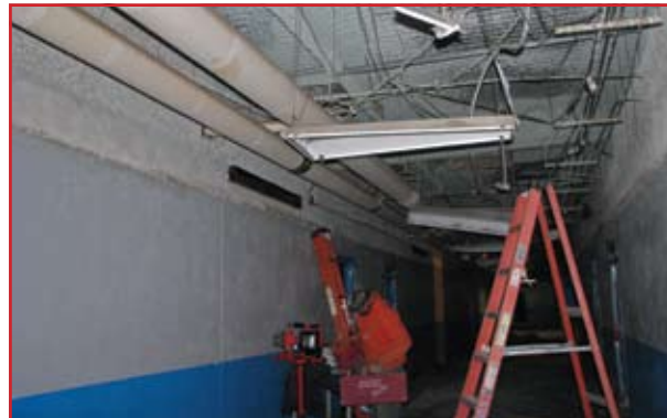
Ceiling tiles removed for access to upgrade electrical and data systems.
