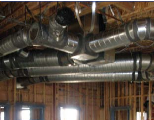
Classroom HVAC ductwork installed and joints sealed; inter-classroom connecting ductwork will complete the installation.
