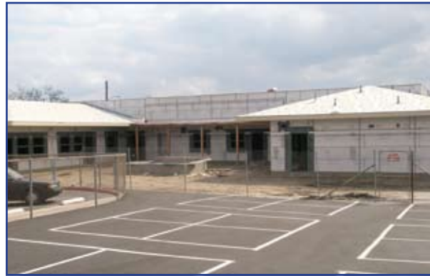
The SDC building overlooks a new portion of the playground area that was rebuilt as part of this project.
