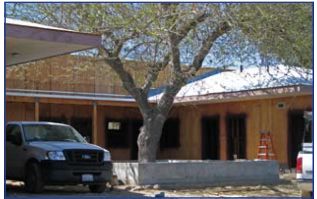
Building exterior to be wrapped with moisture resistant membrane followed by lath and plaster.
