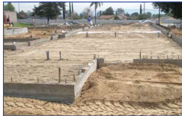
Stem walls poured, utilities stubbed in; slab foundation rebar and cement up next.
