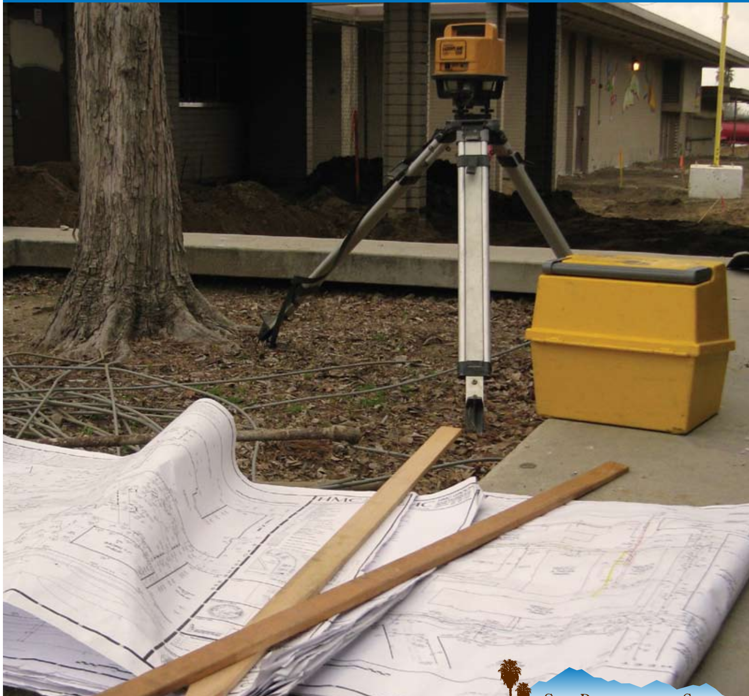
High School #8 New Campus Surveyor's equipment and plans at High School #8, where demolition work has begun.
