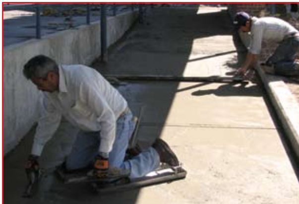
Fairfax ES Workers hand trowel cement finishwork for new ADA-compliant ramps.
