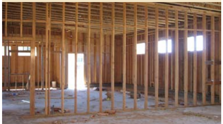
Rough carpentry includes framework, exterior walls and roof.
