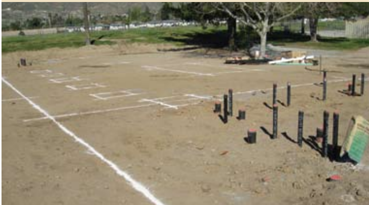
Underground utilities stubbed out; ground marked for excavation of foundation.
