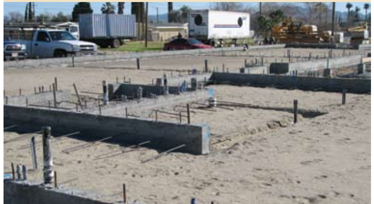
Foundation concrete in place; next is foundation floor concrete pours.
