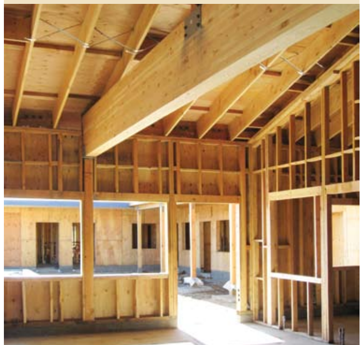
Rough framework complete, building enclosed; massive support beams carry weight of roof.
