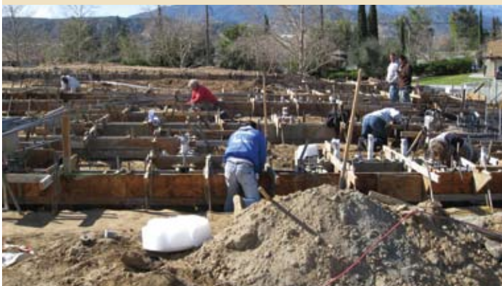
Ground excavated; concrete formwork and rebar going into place for foundation pours.
