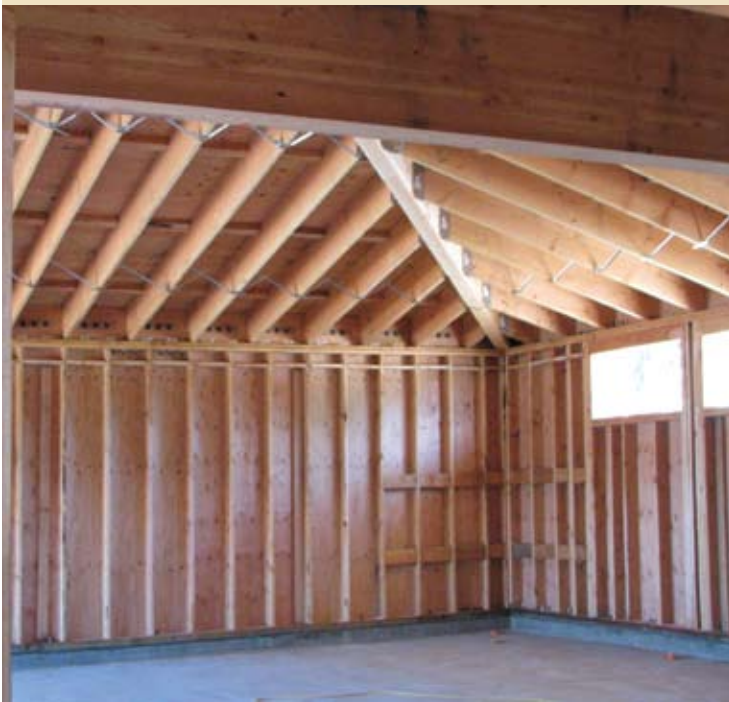
Rough framing complete, structure enclosed, ready for electrical and HVAC conduit installation.
