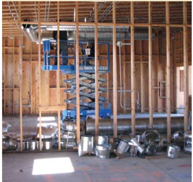
Electrical conduit placed along wall framing; HVAC ductwork suspended from ceiling.
