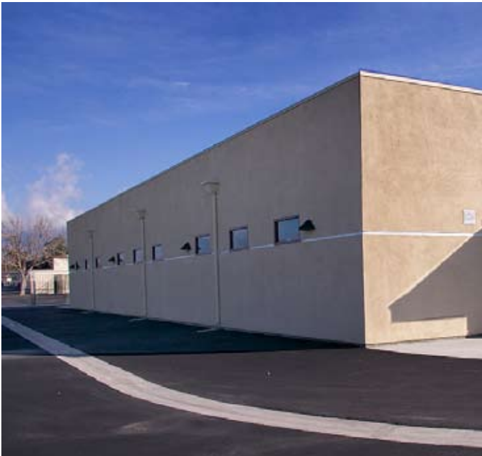
Completed construction of this SDC building included new pavement and storm drainage.
