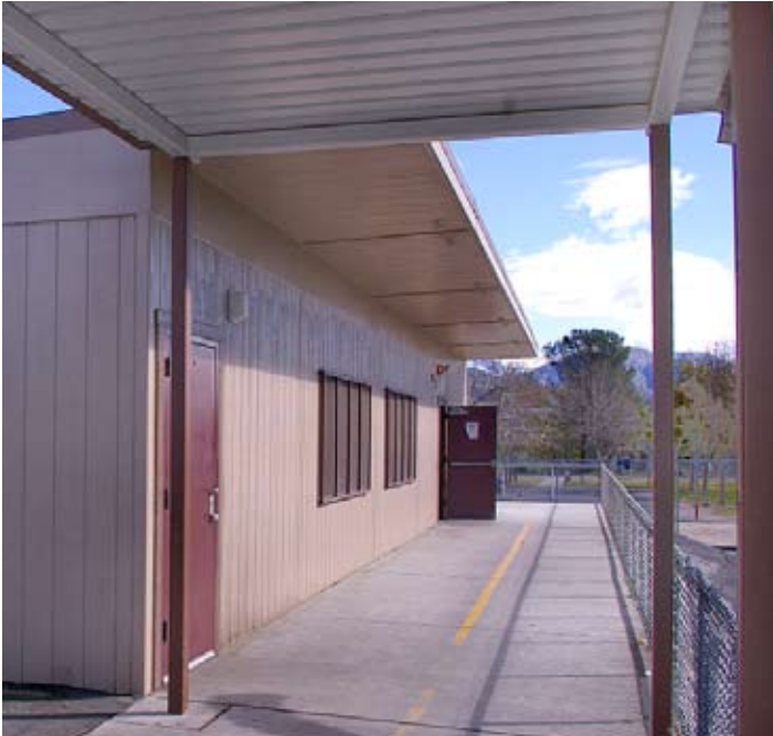
Exterior view of typical multi-use room project with ADA compliant doorway and ramp with fenced railings surrounding the perimeter.
