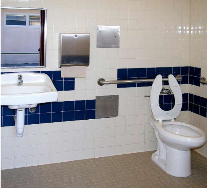
Part of the modernization project budget, new ADA accessible restrooms include new plumbing systems, lighting, wall and floor tiles and water-conserving sinks and toilets.
