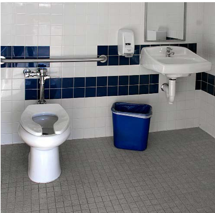
ADA-compliant staff restrooms are included in modernization project's scope of work.
