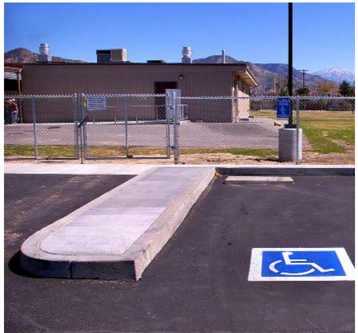
Part II site improvements: ADA-compliant campus entrance and parking lot with ramp, ADA signage, stripping and accessible sidewalks.
