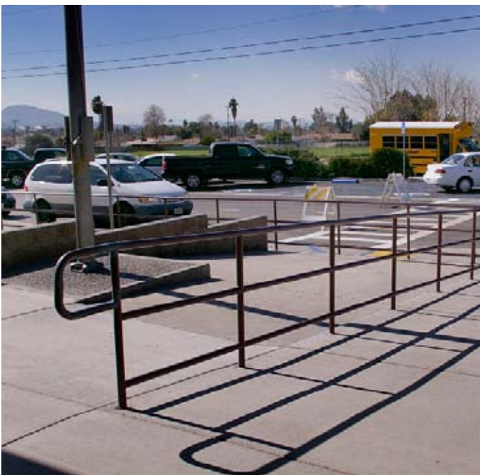
ADA-compliant campus access sidewalks and ramps.
