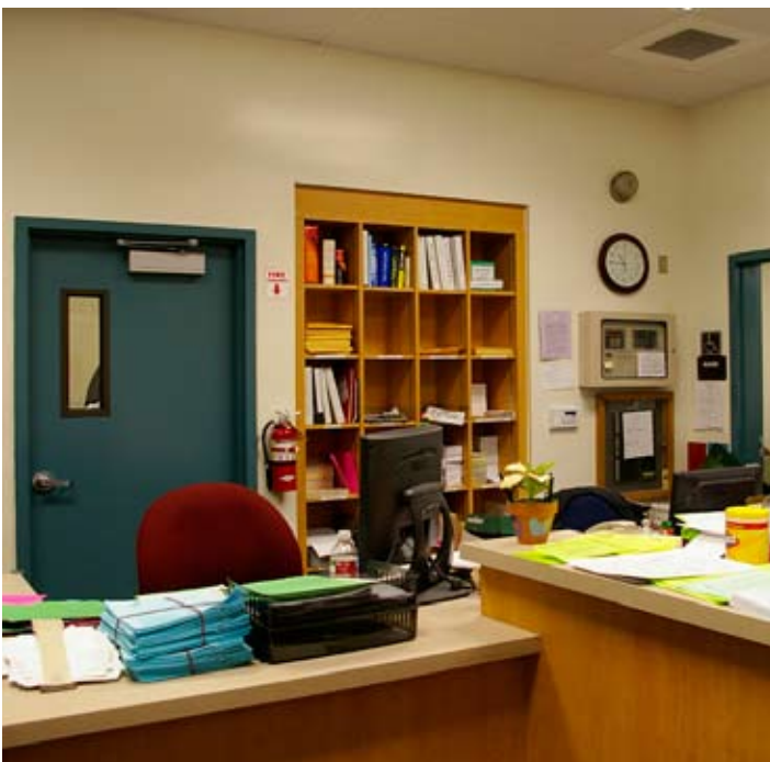
Front office interior upgrades include built-in storage shelving system, cabinets, ADA accessible front desk and counter casework.
