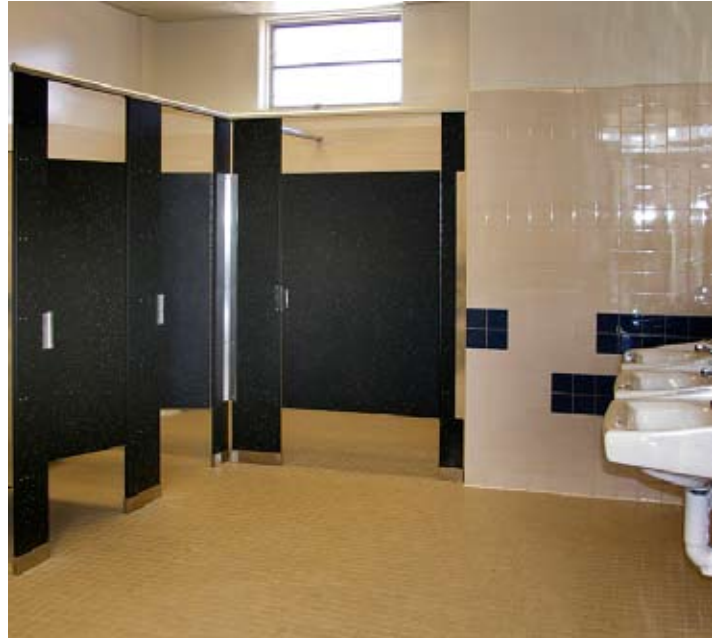
Staff and student restrooms retrofitted with ADA-compliant doors, hardware and signage.
