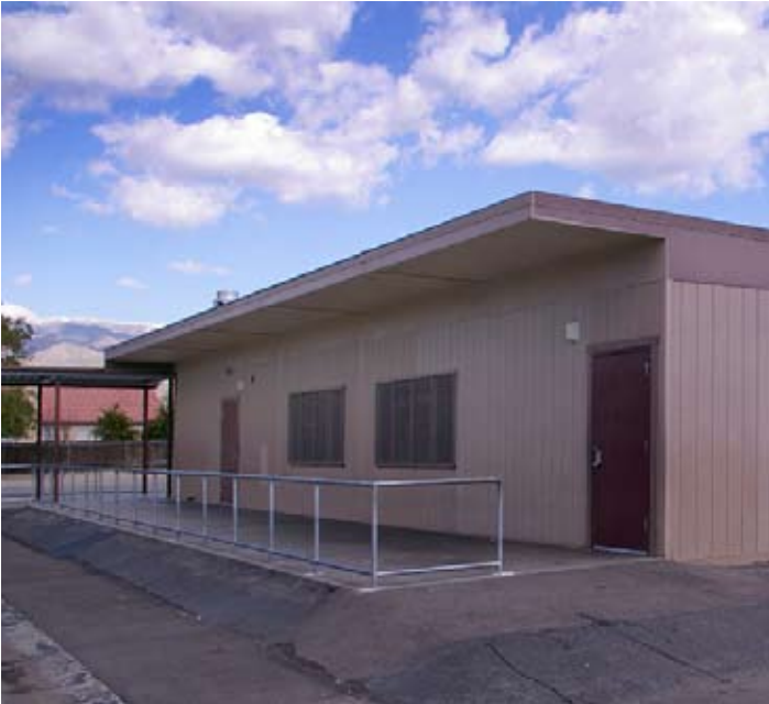
Last phase of the Multi-Purpose room construction concluded with ADA access finish work such as ramp railing shown here.
