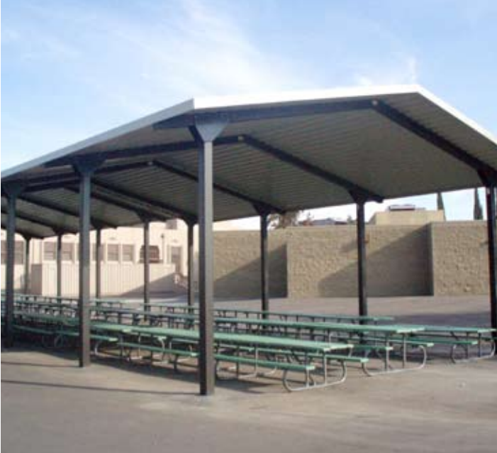
Lunch/shade shelter completed in Fall 2006.
