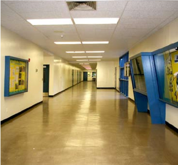
Building A modernized lighting, ceiling, walls; new enclosed offices along left side of corridor.
