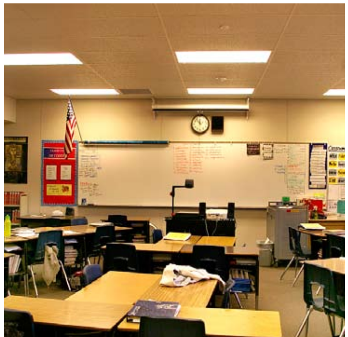
Typical classroom modernizations include: improved lighting, lowered acoustical ceiling, hi-traffic carpeting, tackable wall surfaces.
