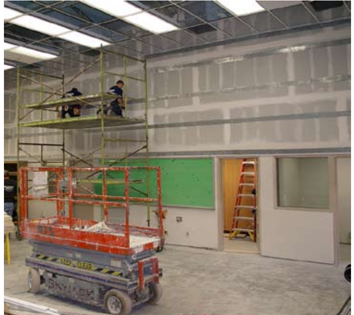
Music and Choir rooms are being outfitted with acoustical ceilings and walls, risers and ADA accessible ramps.
