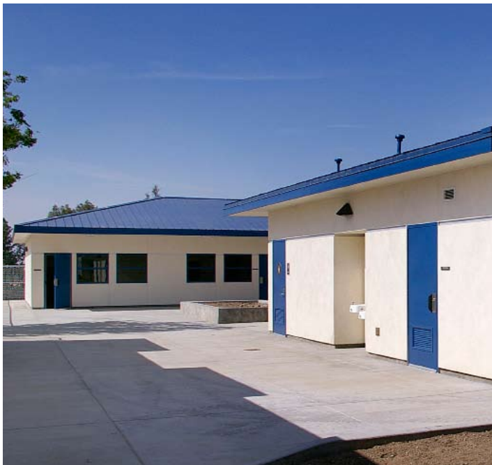
Exterior work complete with concrete planter in center courtyard.
