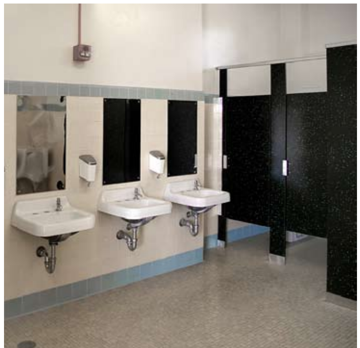
ADA-compliant student restrooms include new plumbing systems, lighting, wall and floor tiles.
