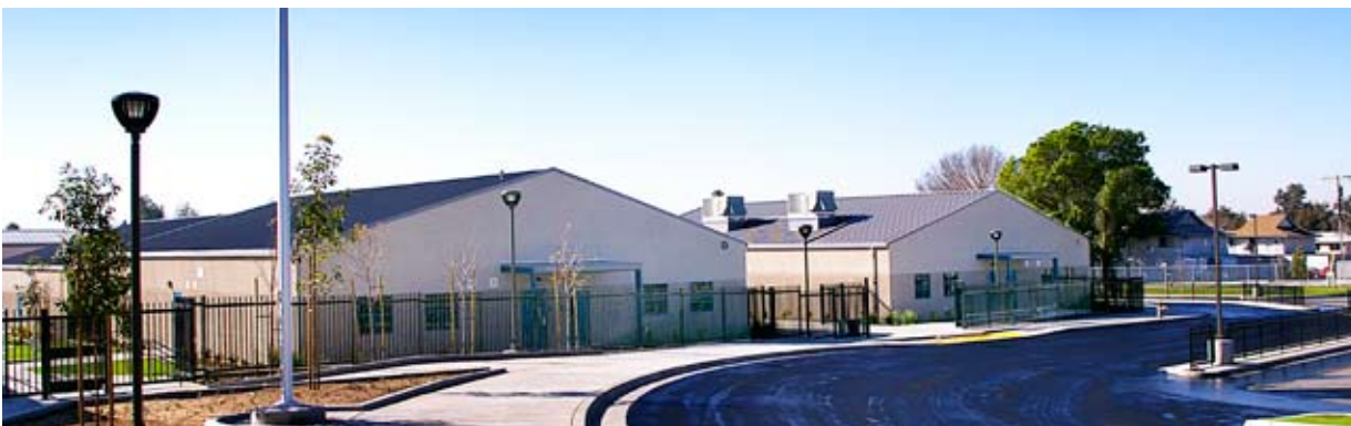
View of D and C classroom buildings from north campus bus and vehicle area. Staff parking is located on the far right.
