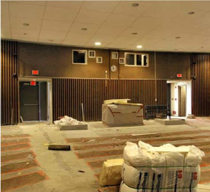
New lighting, raised acoustical ceilings, carpet, seating, stage lighting, and sound systems as well as ADA access upgrades will complete this student theatre.
