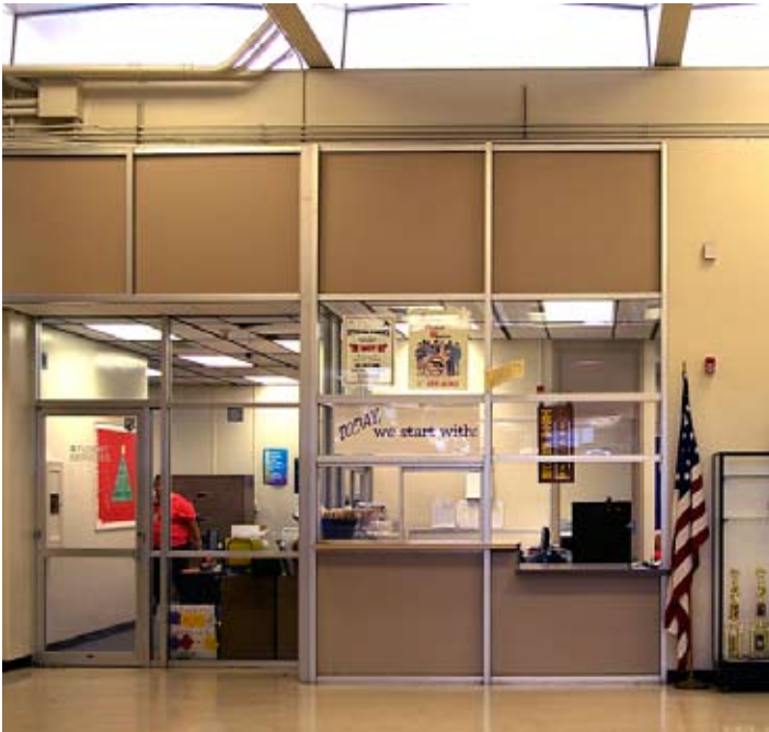
Newly remodeled School Office with ADA accessible service window, new lighting and ceiling, new paint and reconfigured office walls.
