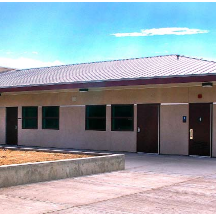
District standards require exterior paint of completed buildings coordinate with school colors for all SDC buildings.
