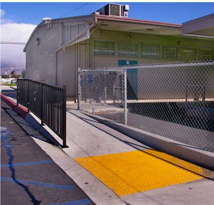
Finish work for Multi-Purpose room construction included installation of ADA-compliant access to the campus.
