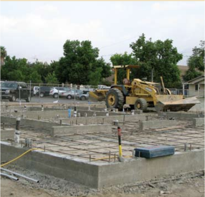
Concrete foundation walls poured, rebar being place for concrete foundation slab pour.
