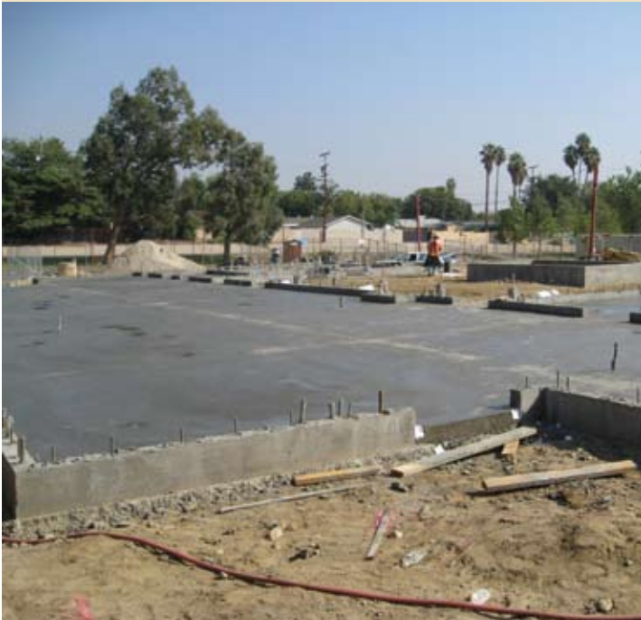
Concrete foundation slab poured; once concrete is cured, structural framework goes up.
