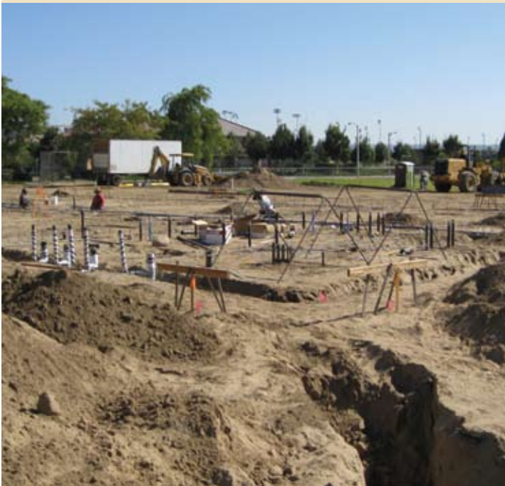
Utilities stubbed out; trenching for foundation walls is underway; formwork to follow.
