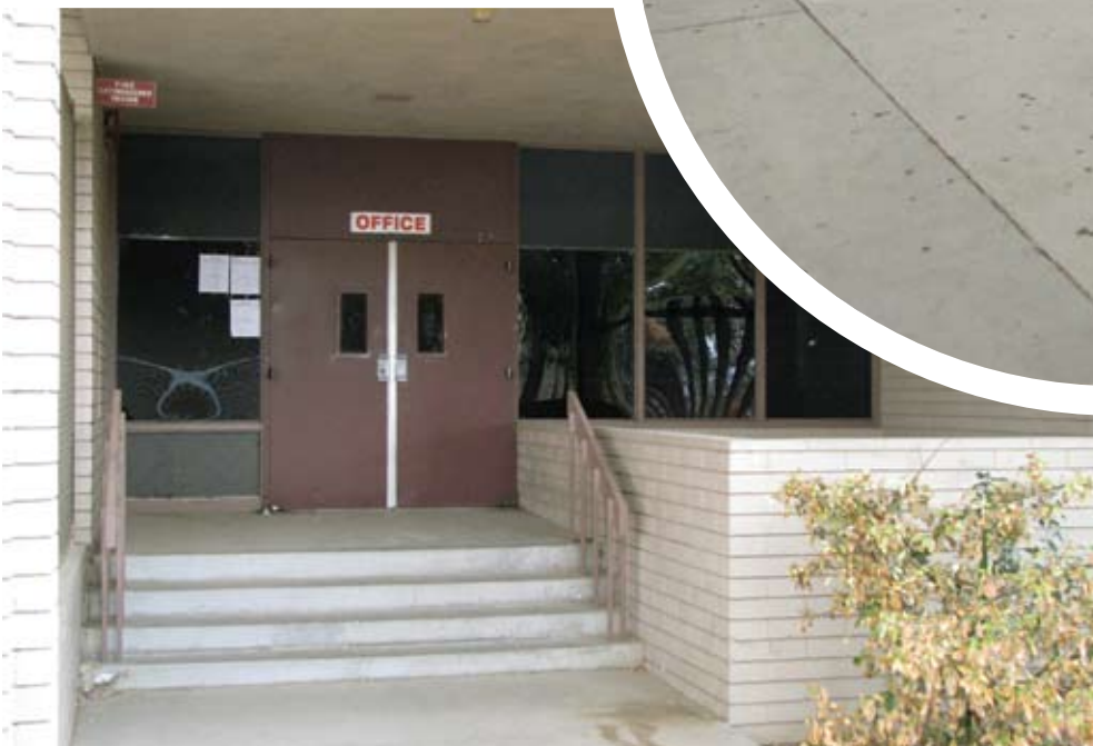
Right Existing front office and administration building to be modernized and repurposed as classrooms, faculty center and food lab.
