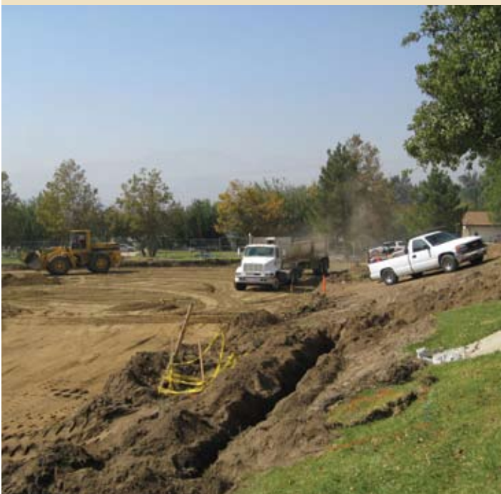
Sitework includes grading into hillside and trenchwork for underground utilities and foundation.
