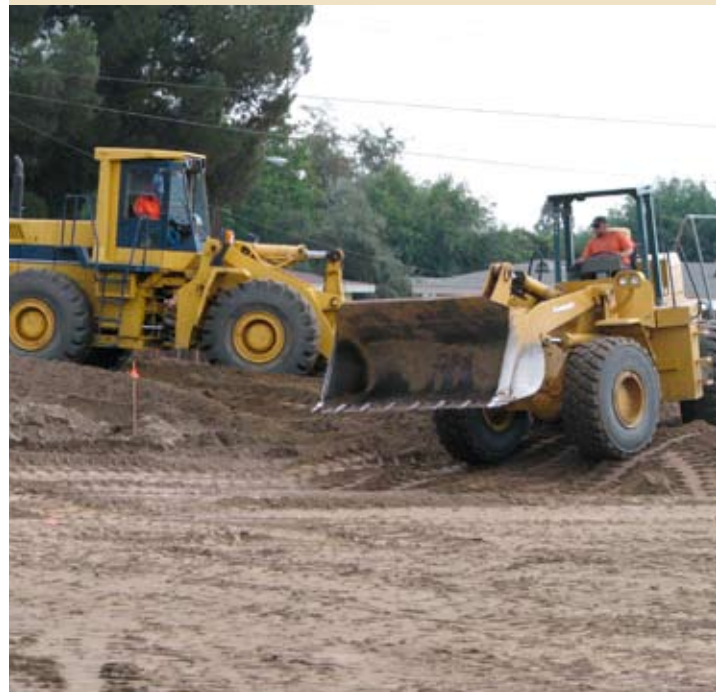
Initial sitework includes earthwork and grading.
