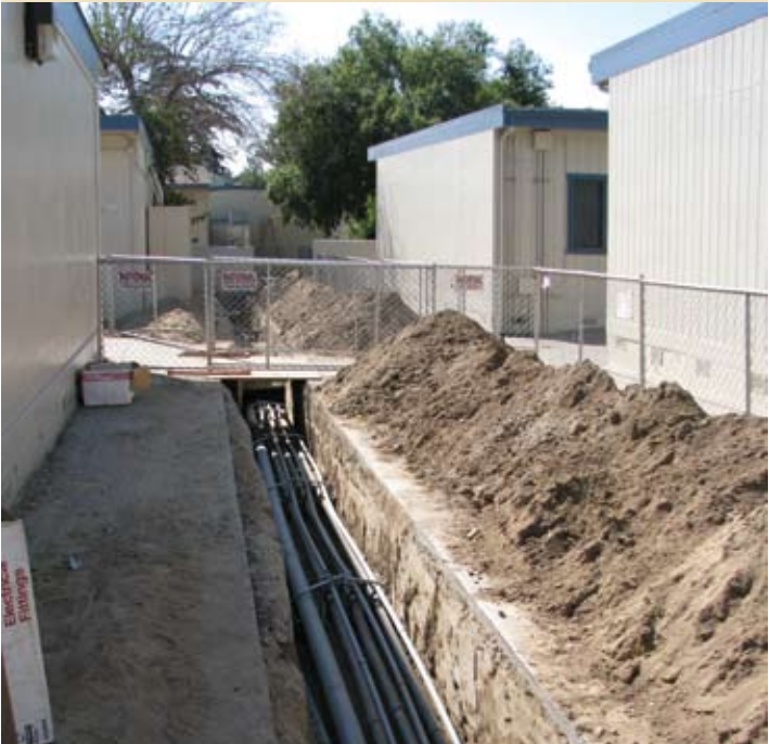
Tie-in of existing underground utilities involves trenching and extending from the main campus to the SDC site at the north end of campus.
