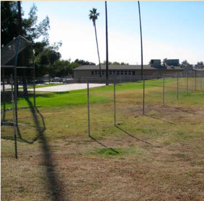
Temporary fencing of construction site installed; contractor staging area to be located in parking lot.
