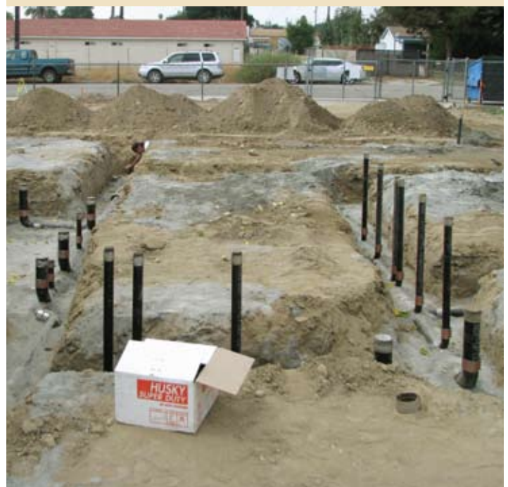
Site graded, underground utilities trenched with stubouts.
