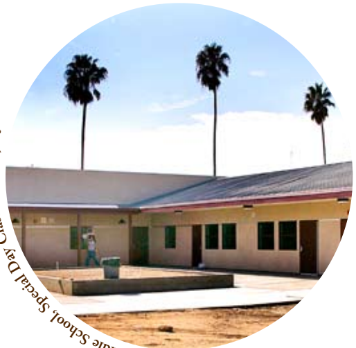
Arrowview Middle School, Special Day Classroom Project
