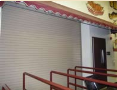
San Andreas High School, Kitchen Upgrade
