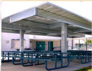
Palm Ave Elementary School, Lunch Shelter
